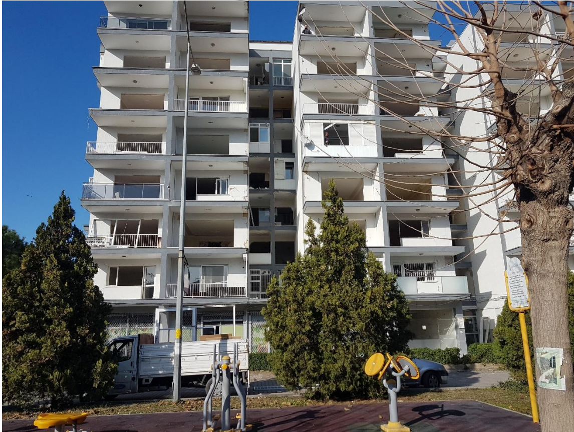
Figure 1 Pre-Demolition View of the HK 6 Project Building
