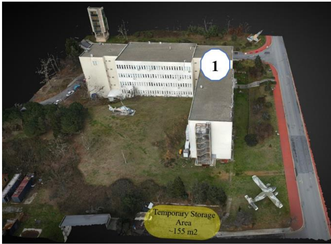
Figure 3: ITU Ayazağa Campus Faculty of Aeronautics and Astronautics Building Temporary Storage Area
