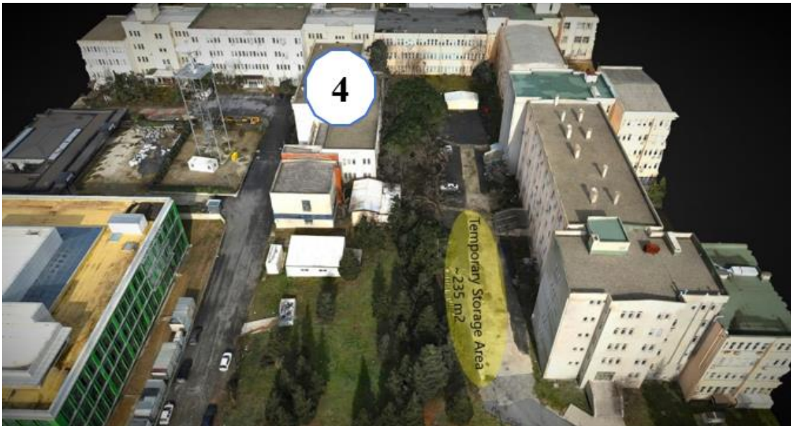
Figure 5: ITU Ayazağa Campus Faculty of Mining Engineering Building Temporary Storage Area
