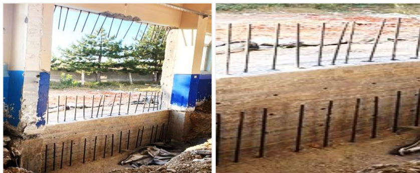
Figure 11: EXAMPLE VISUAL OF ANCHORAGE BARS BEING DRIVEN
