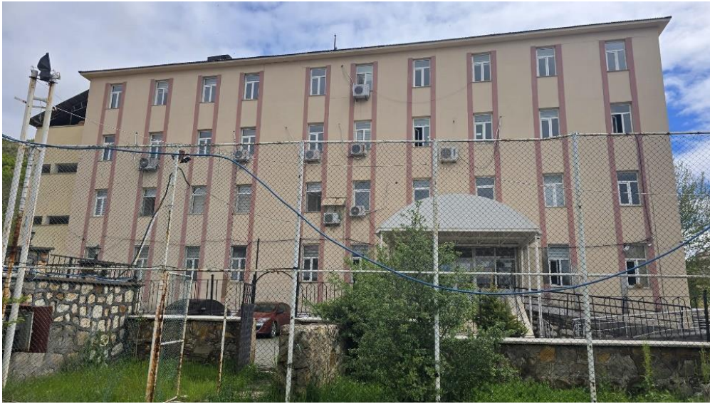
Figure 8 - Nazimiye Government House General View - 4
