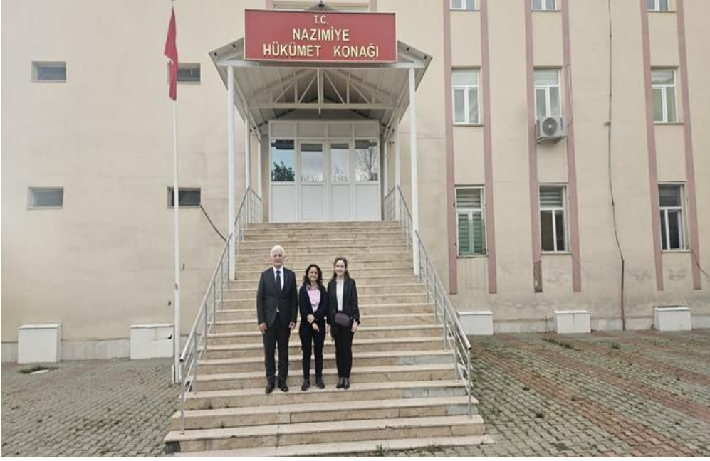
Figure 7 - Nazimiye Government House General View - 3
