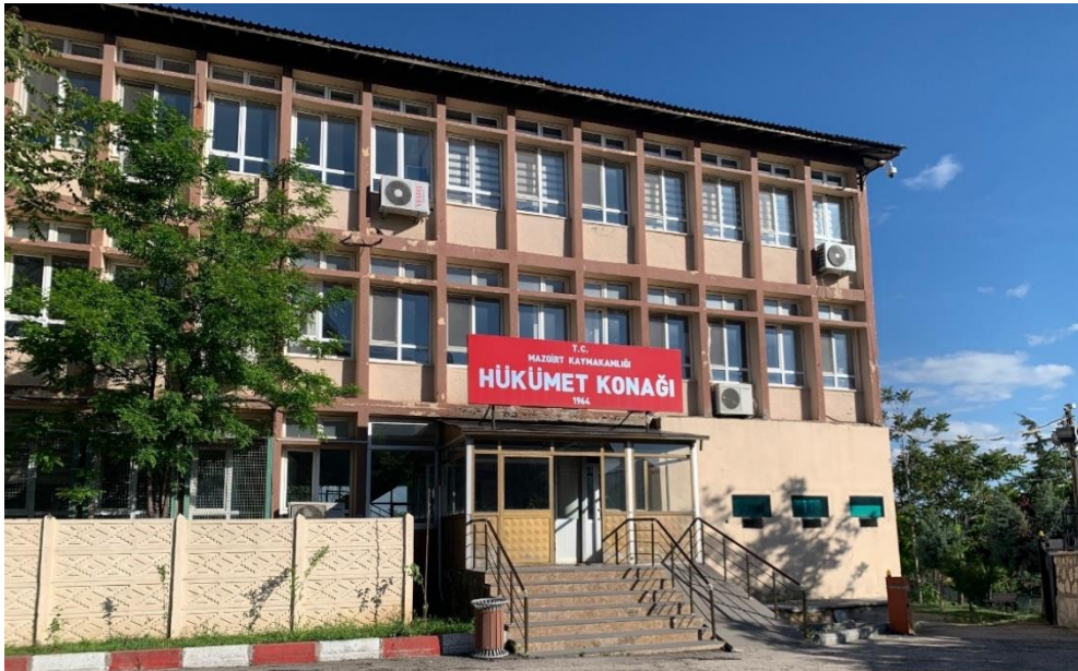
Figure 6 - Mazgirt Government House General View / 2
