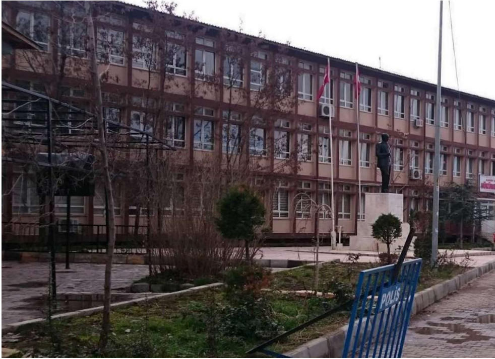
Figure 5 - Mazgirt Government House General View
