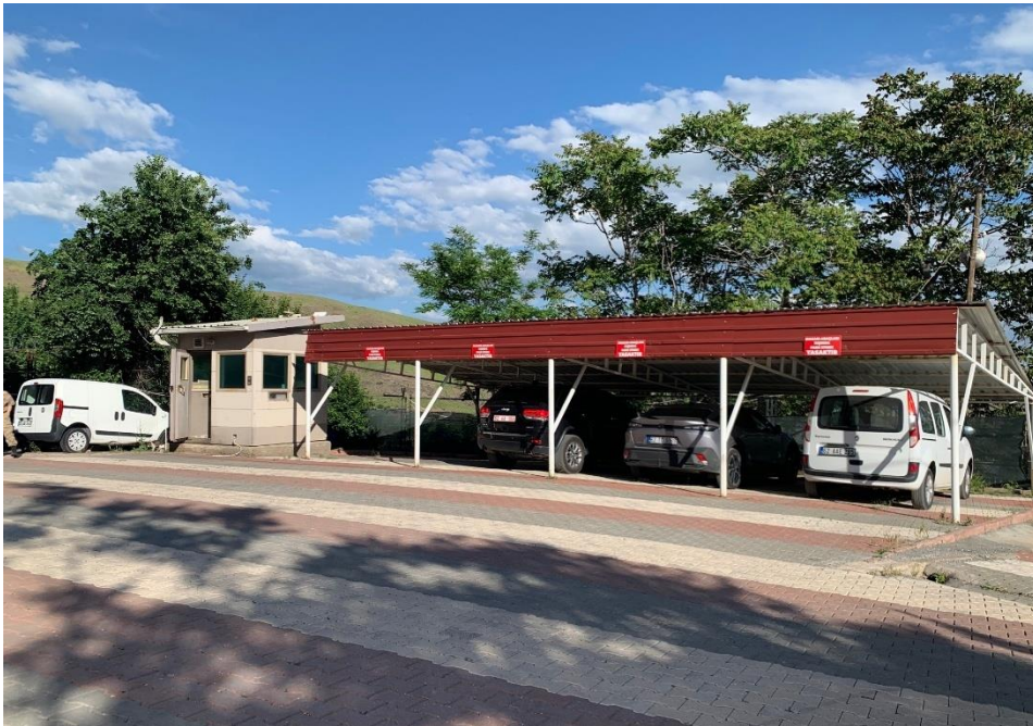
Figure 8 - Mazgirt Government House Backyard
