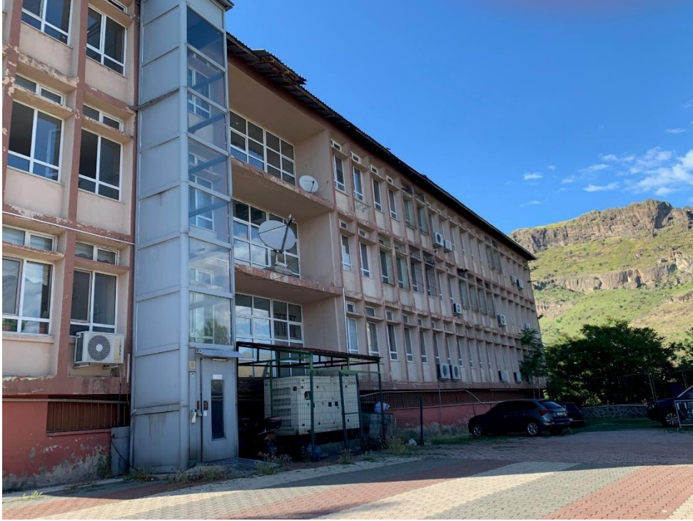
Figure 7 - Mazgirt Government House Back View
