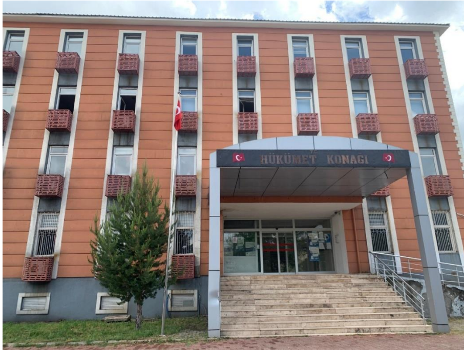
Figure 5 - Hozat Government House General View /1
