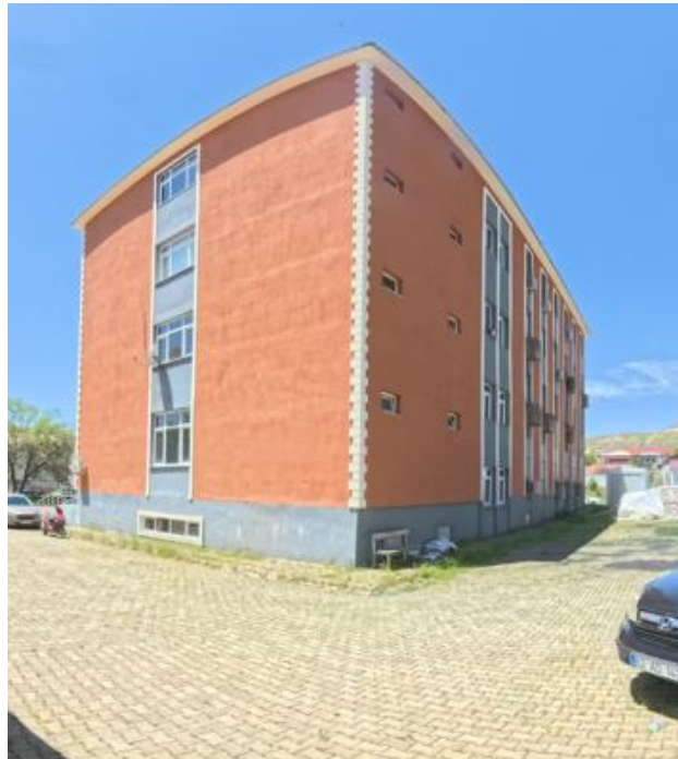
Figure 6 - Hozat Government House General View /2
