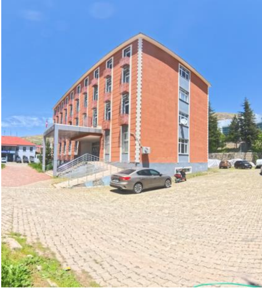
Figure 7 - Hozat Government House General View /3
