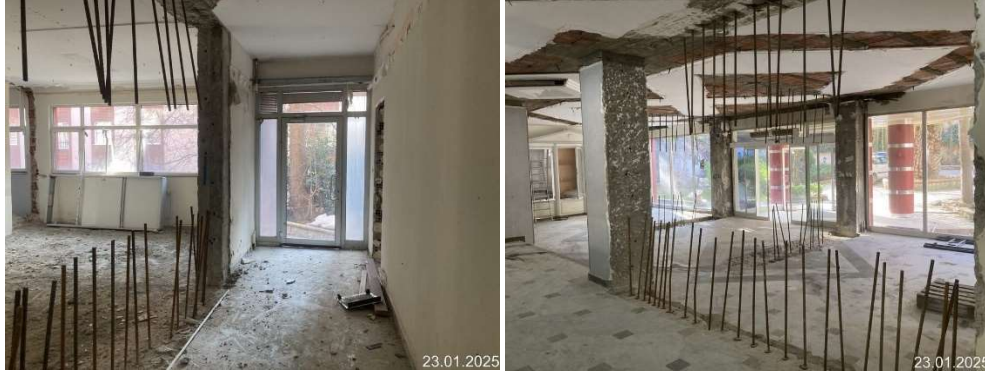
Figure 20 - Sample Image of Anchor Bar Installation
