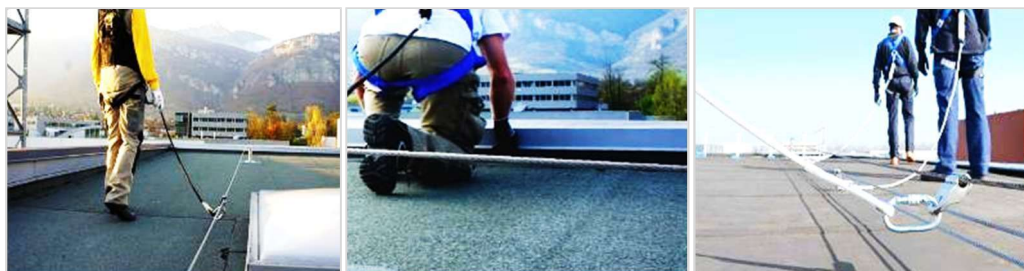
Figure 12 - Representative Image of a Movement Restraint System
