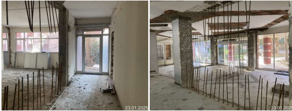
Figure 9 - Sample Image of Anchor Bar Installation
