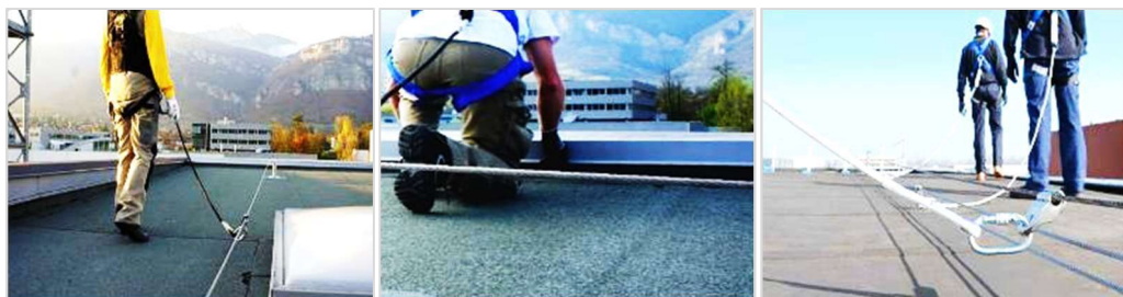
Figure 12 - Representative Image of a Movement Restraint System
