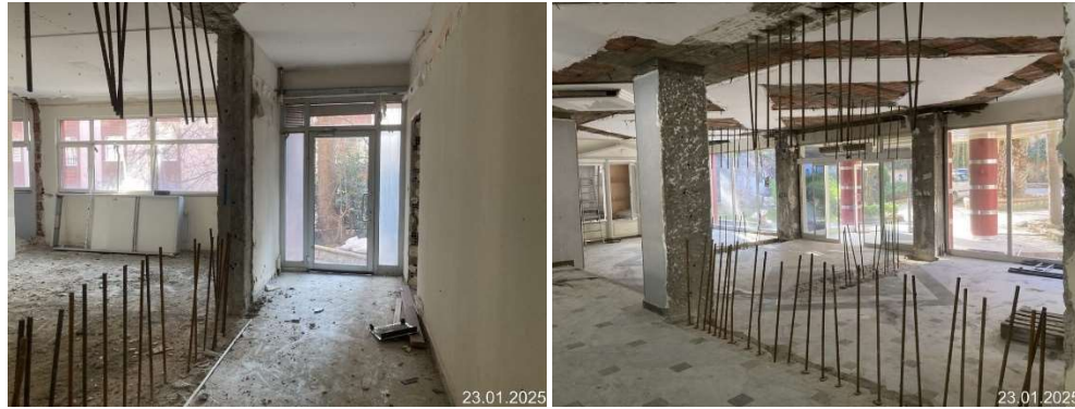
Figure 9 - Sample Image of Anchor Bar Installation
