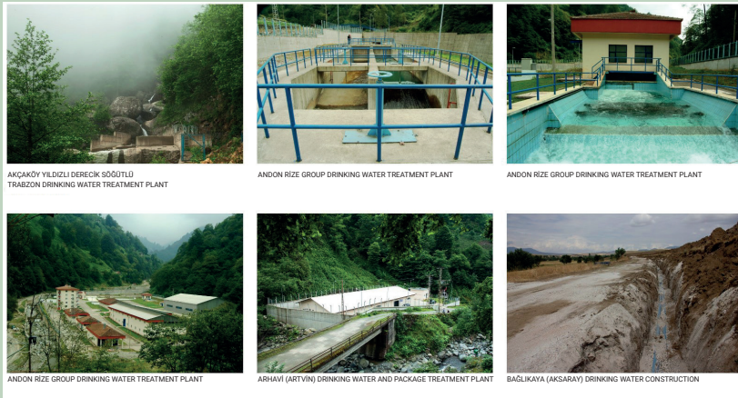
Drinking Water Facilities Constructed by İLBANK
