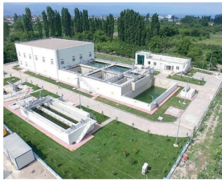
İZNIK (BURSA) MBR TECHNOLOGY WASTEWATER TREATMENT PLANT
