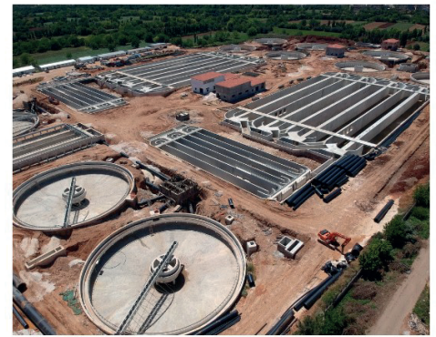
GAZİANTEP GASKİ CENTRAL TREATMENT PLANT
