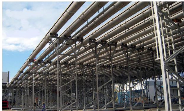
Figure 6. First commercial application of g 3 technology in 2009 – transmission lines in Jebel Ali (UAE)
