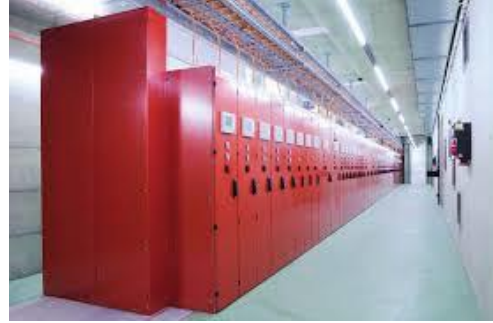
Figure 9. Images of 170 kV HV GIS and 24 kV MV GIS equipment installed in pilot substation shown in Figure 8
