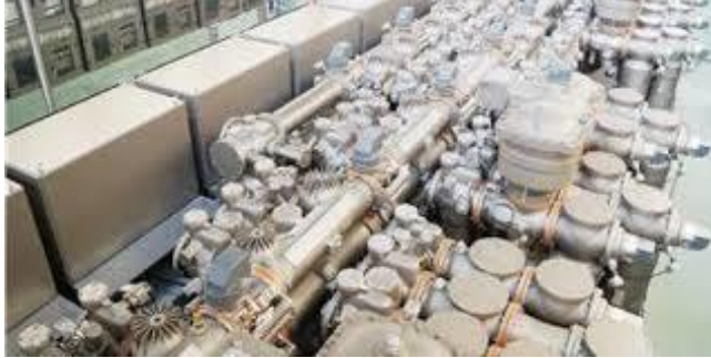
Figure 9. Images of 170 kV HV GIS and 24 kV MV GIS equipment installed in pilot substation shown in Figure 8
