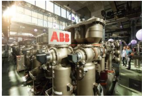
Figure 8. A pilot substation in Oerlikon (Switzerland) where HV GIS 170 kV and MV 24 kV equipment that uses ABB proprietary gas insulating mixture containing Novec 5110™ was installed.
