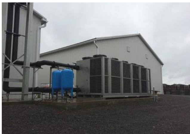
Figure 8: Indirect system using HC refrigerant
