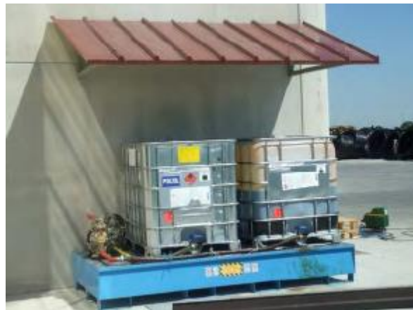
Figure 6 IBC tanks with pre-blended polyol containing cyclopentane
