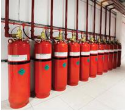
Figure 4. Examples of total flooding systems where Novec 1230™ is used
