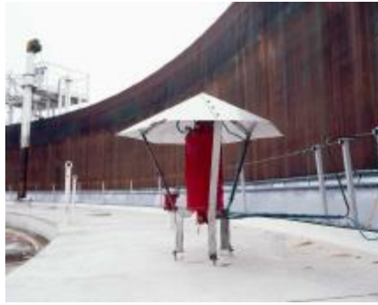
Figure 7. Floating roof tank protected by CF_3I – based fire extinguishing system.
