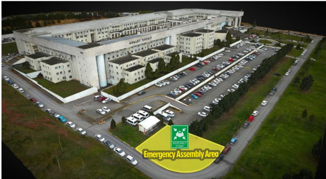
Figure 14: Sakarya Government Office Emergency Assembly Area
