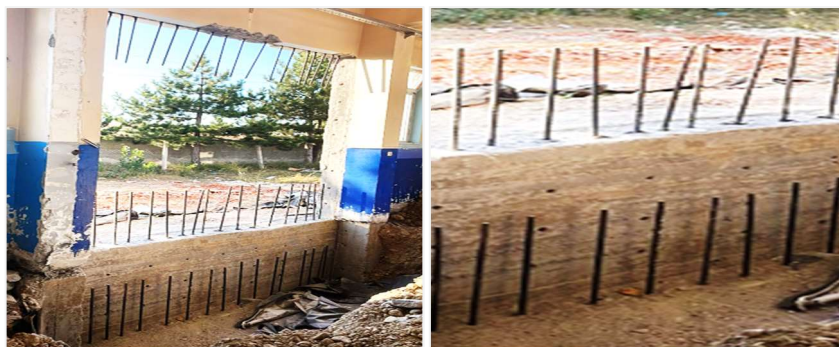
Figure 10: Installing Anchor Rods Sample Image
