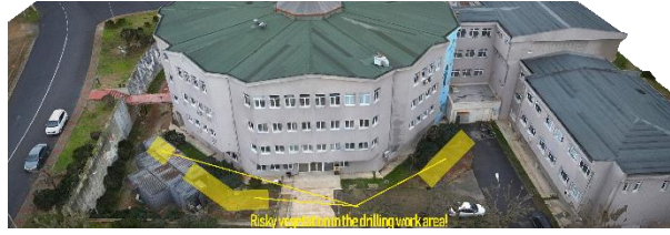
Figure 9: RISKY VEGETATION AROUND SFLA BLOCK
