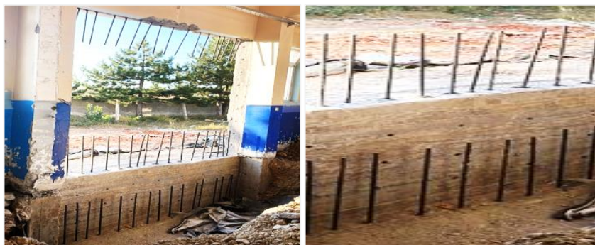
Figure 7: Installing Anchor Rods Sample Image
