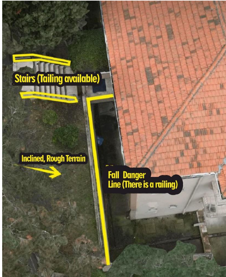
Figure 16 BOĞAZIÇI UNIVERSITY KANDİLLİ CAMPUS NEW GEOPHYSICS BUILDING Risky Areas
