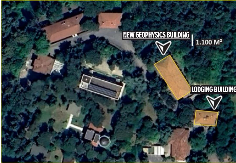
Figure 1 BOĞAZIÇI UNIVERSITY KANDİLLİ CAMPUS NEW GEOPHYSICS BUILDING (Campus No: 1)
