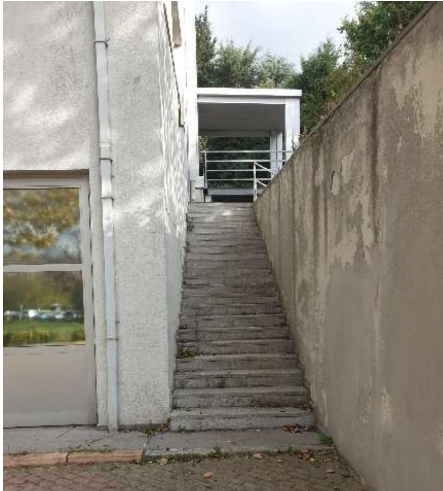
Figure 19 Ladders without appropriate guardrails
