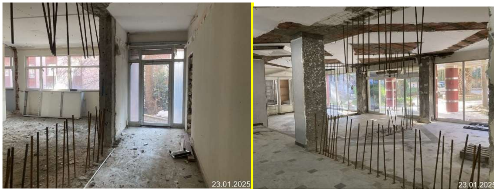
Figure 14 Sample Image of Anchor Bar Installation
