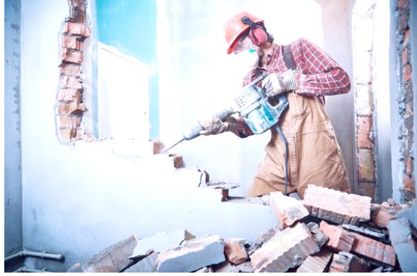
Photo 11: WALL DEMOLITION SAMPLE IMAGE
