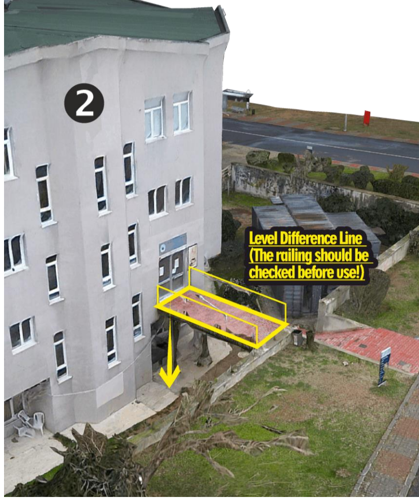
Figure 10: BOĞAZIÇI UNIVERSITY KILYOS CAMPUS BUILDING 2 LEVEL DIFFERENCE WARNING (FALL RISK)
