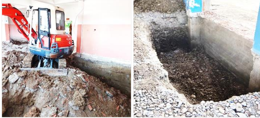
Photo 12: OPENING AROUND THE COLUMN AND SHEAR WALL MANTLE SAMPLE IMAGE
