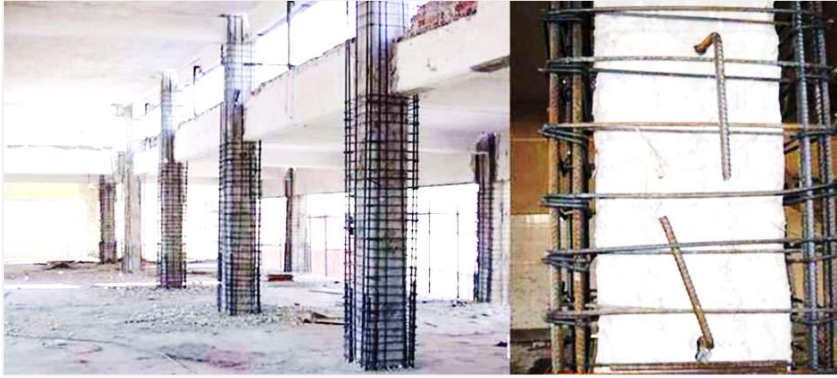
Photo 14: SAMPLE IMAGE OF INSTALLING REINFORCEMENT ELEMENTS
