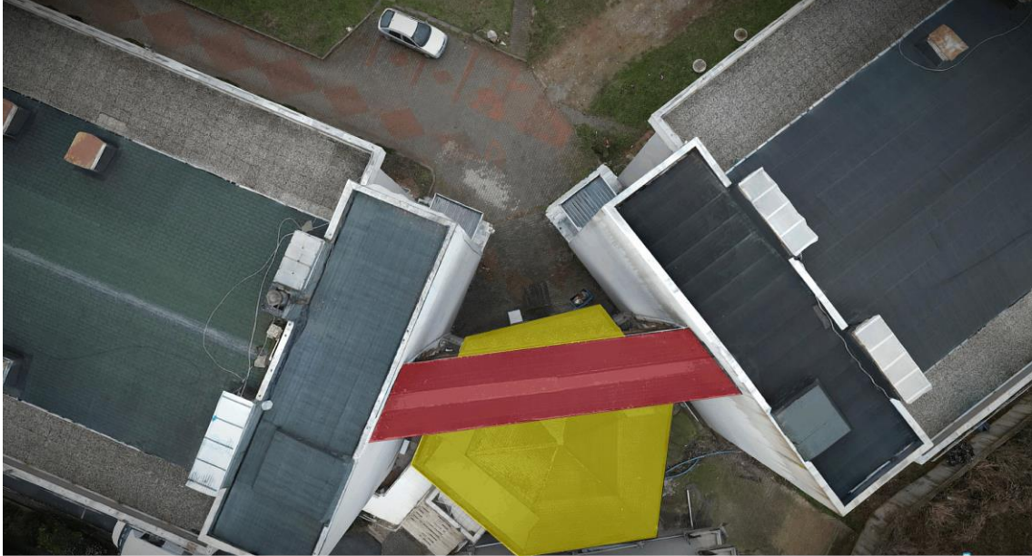
Photo 16: UNDER METAL BRIDGE C BLOCK LOCATION
