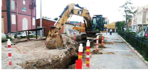
Photo 8 EXCAVATION WORK SAMPLE IMAGE
