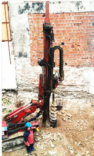
Photo 2: DRILLING EXAMPLE WITH MINI DRILLING MACHINES
