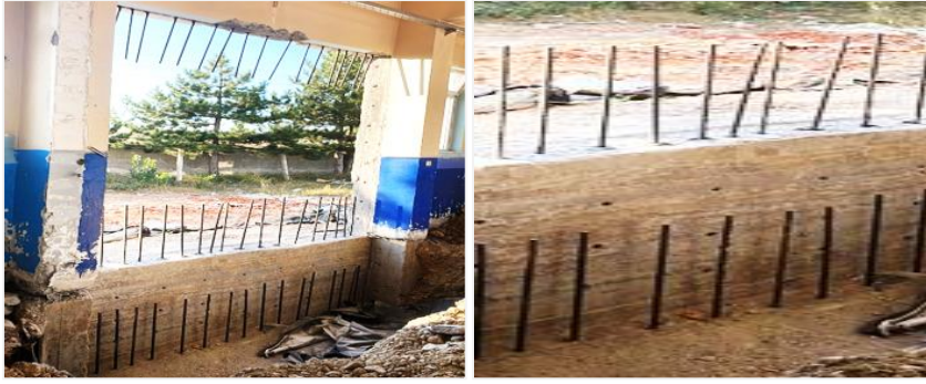
Photo 13: INSTALLING ANCHOR RODS SAMPLE IMAGE
