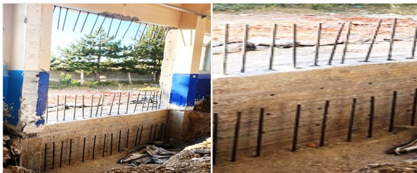
Figure 9: Installing Anchor Rods Sample Image
