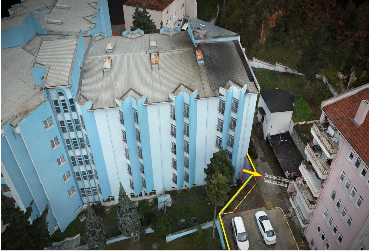
Figure 17 : Gazanfer Bilge Student Dormitory Campus Level Difference Warning (Fall Risk)
