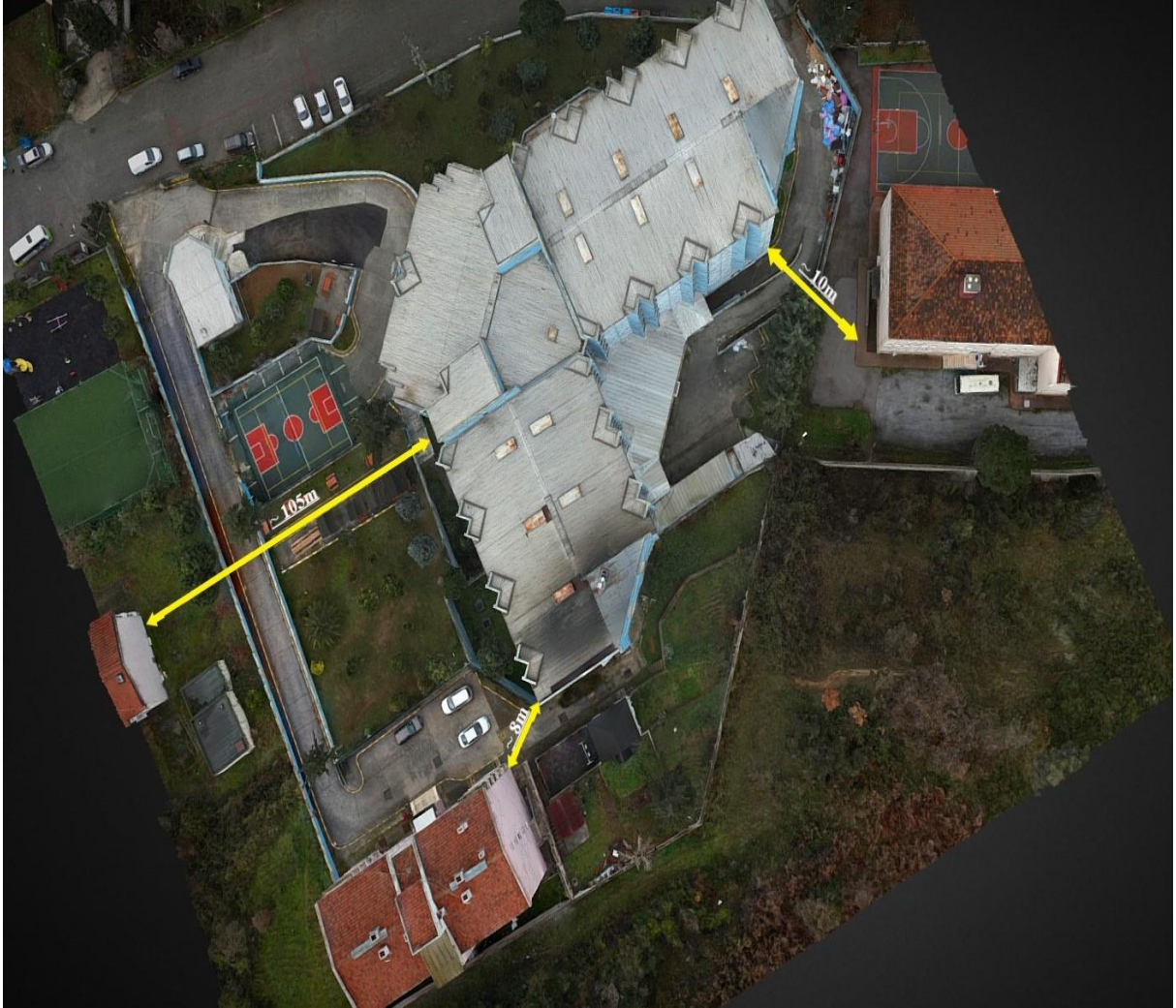
Figure 20 : Gazanfer Bilge Student Dormitory Campus Buildings And Approach Limits
