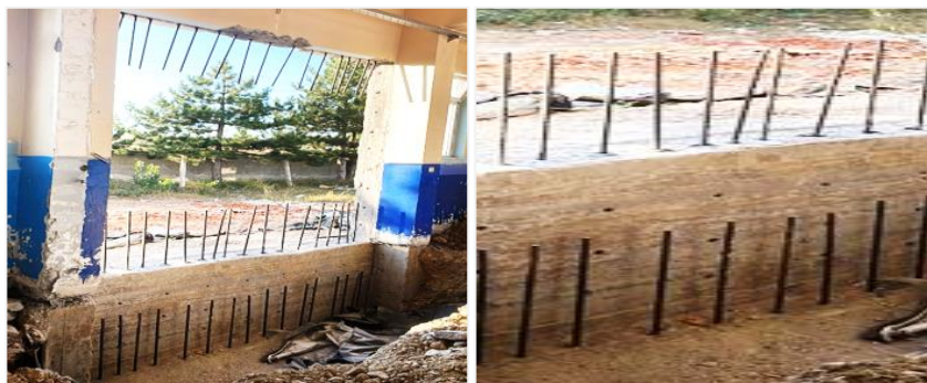
Figure 7: Installing Anchor Rods Sample Image
