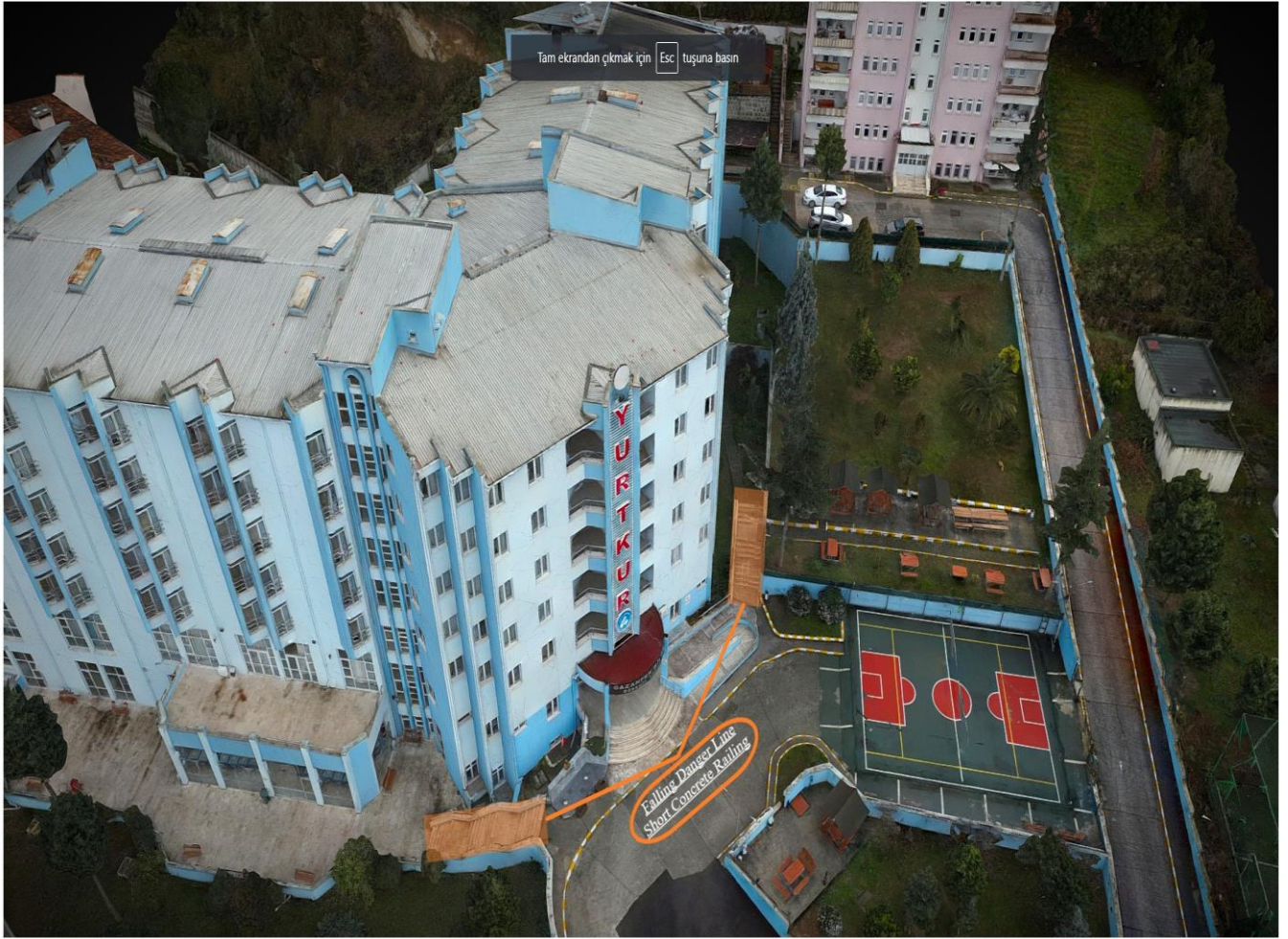
Figure 18 Gazanfer Bilge Student Dormitory Campus Level Difference Warning (Fall Risk)
