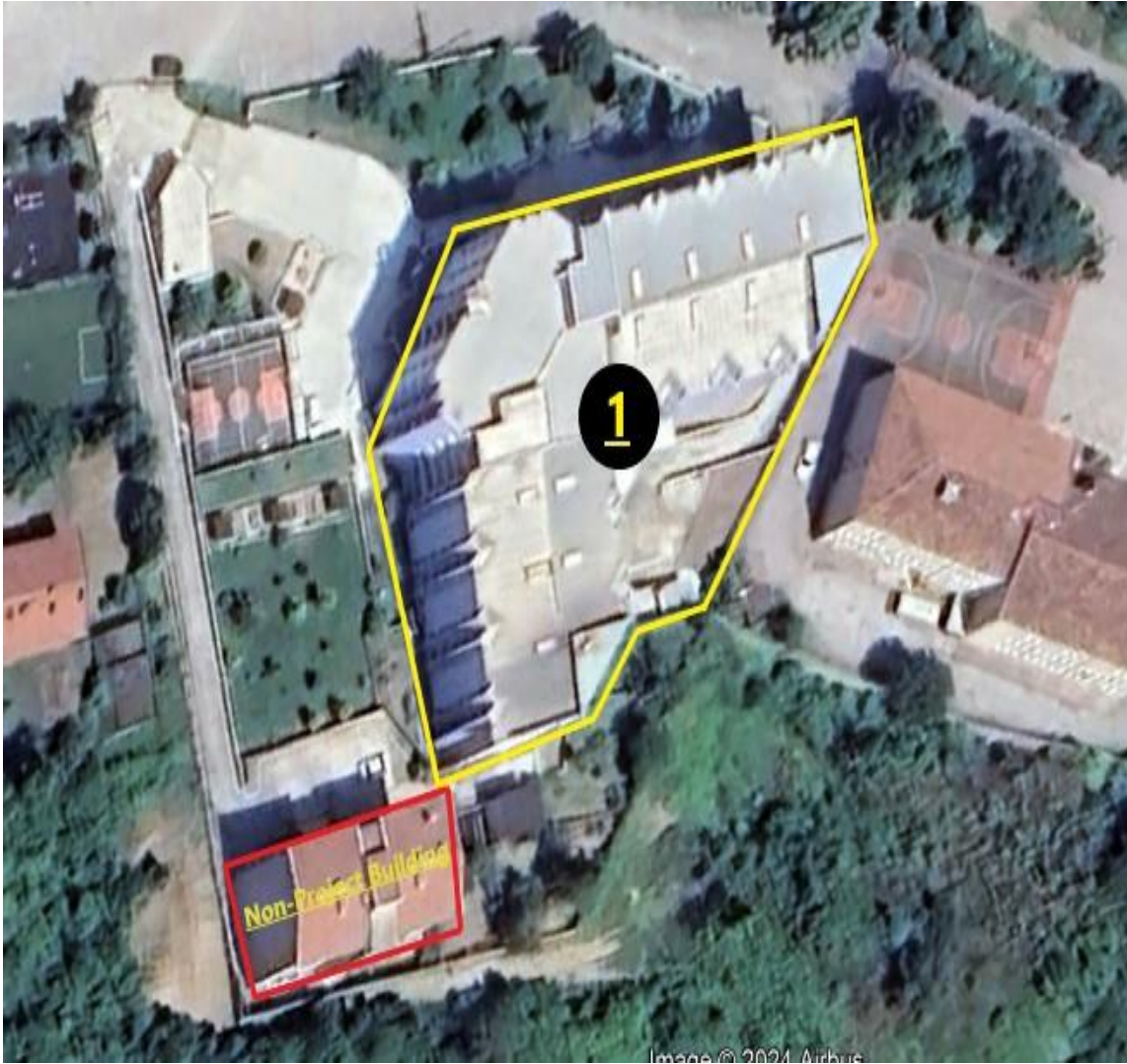
Figure 1 Kocaeli Karamürsel Gazanfer Bilge Student Dormitory (Campus No: 5)
