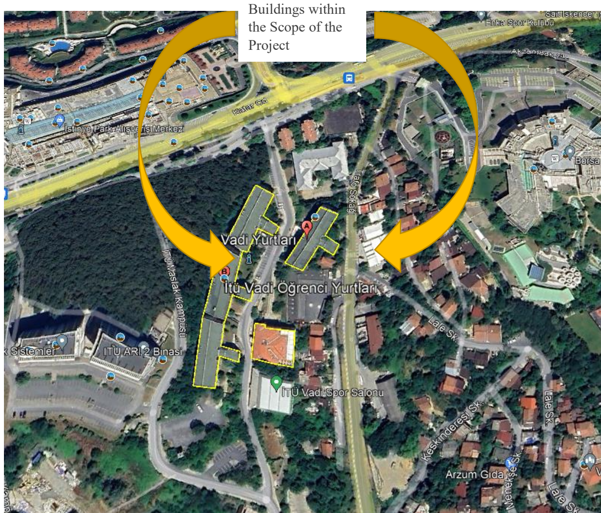
Figure 1: BUILDINGS INCLUDED IN THE SCOPE OF ITU AYAZAGA CAMPUS VADI SECTION PROJECT
