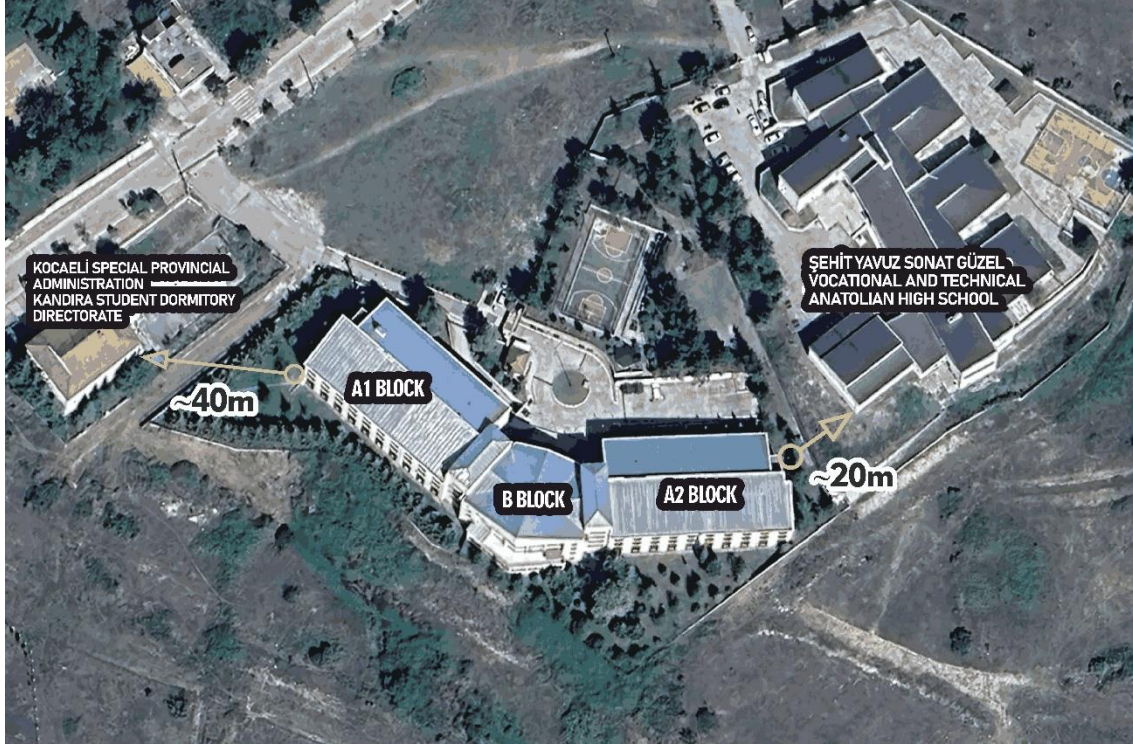
Figure 1-3: Kandıra Girls' and Boys' Dormitory Building View and Coordinates
