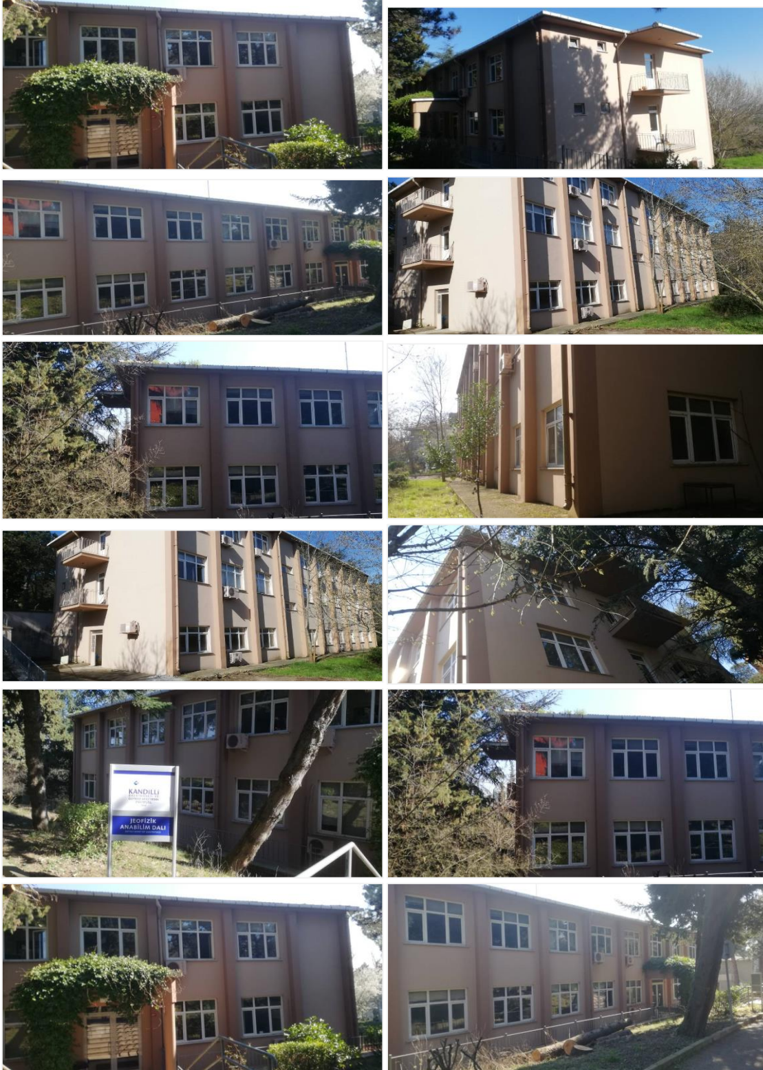
BOĞAZIÇI UNIVERSITY KANDİLLİ CAMPUS NEW GEOPHYSICS BUILDING FACADE PHOTOS
