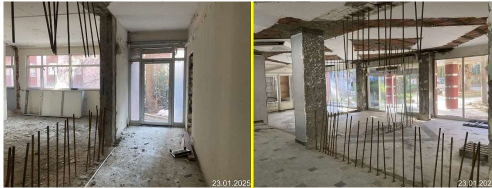
Figure 17 - Sample Image of Anchor Bar Installation
