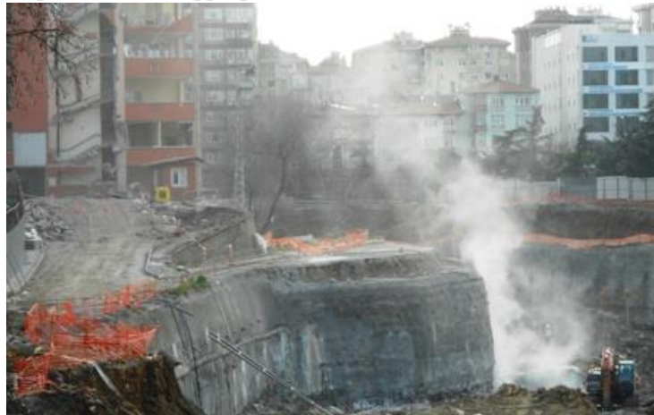
Figure 7 Spread of Dust Generated During the Drilling Operation
