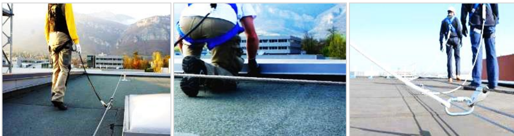
Figure 12 Representative Image of Movement Restrictor (Fall Preventer)
