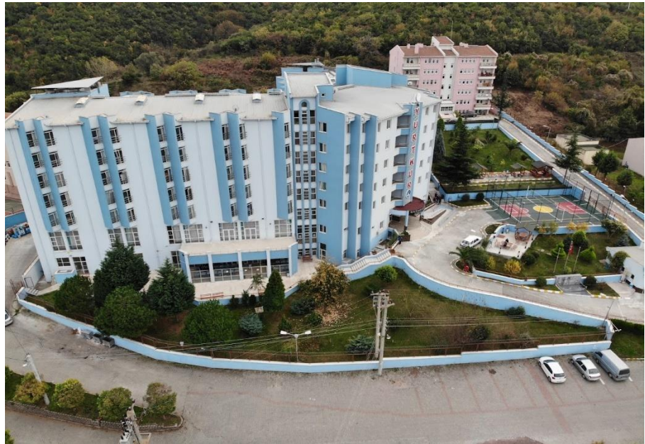
Figure3-2: Gazanfer Bilge Student Dormitory View
