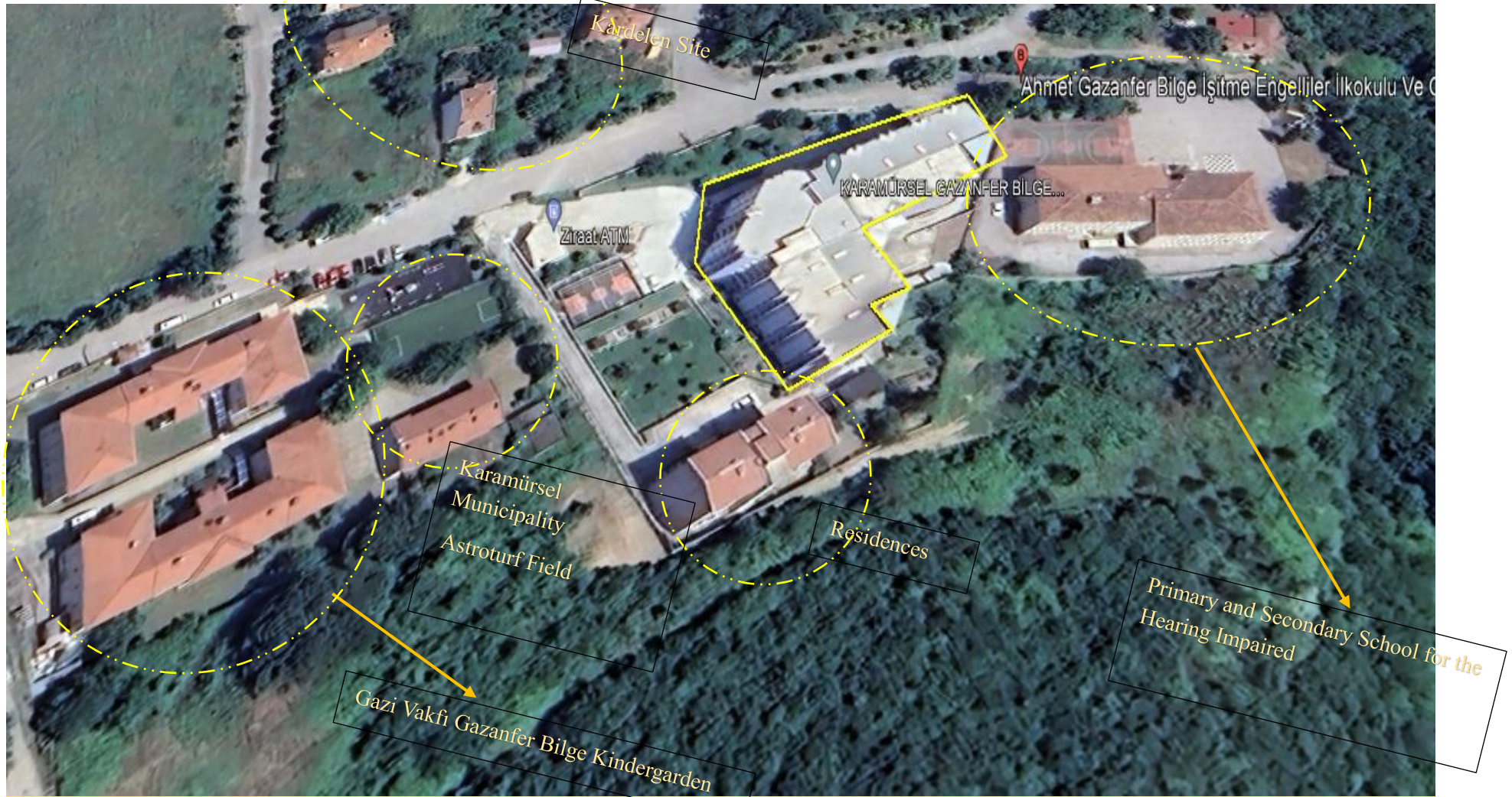
Figure1-4: Approach Distances and Major Impact Area of the Buildings Included In The Scope of the Project
