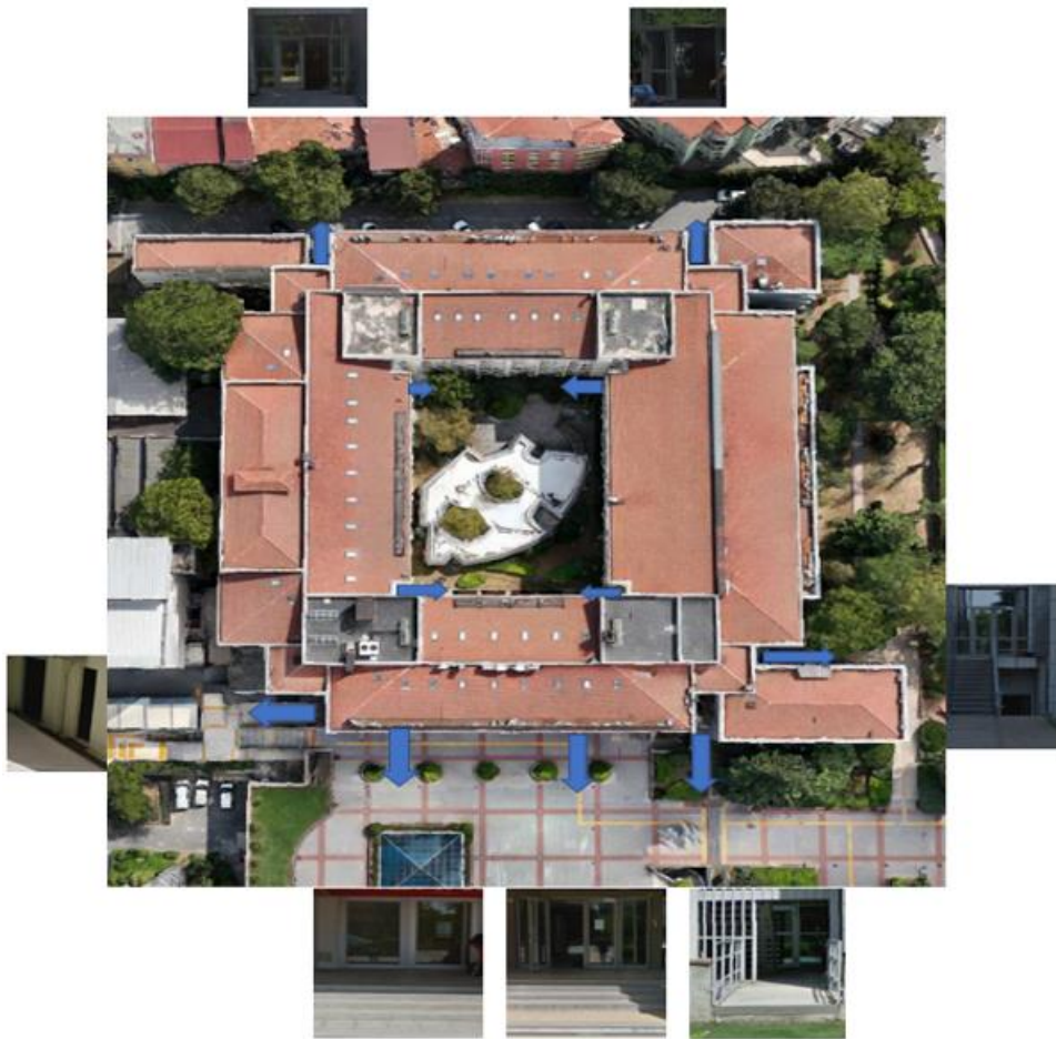
Figure 4: Building Exterior Doors
