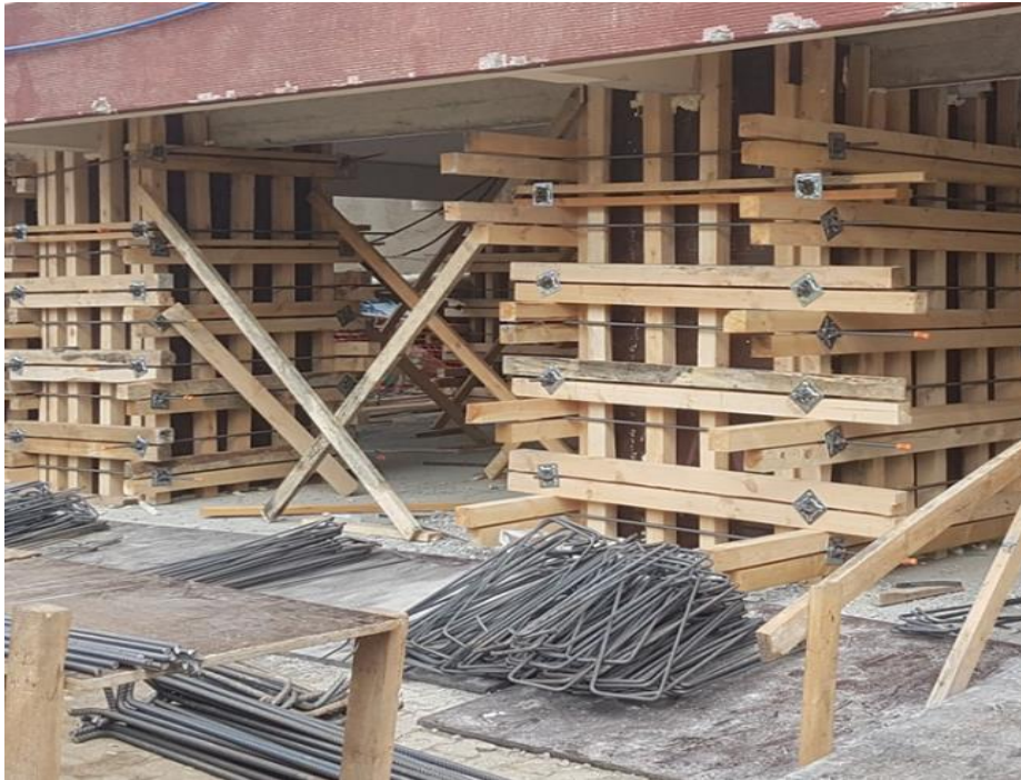
Figure 6: SAMPLE COLUMN JACKETING APPLICATION
