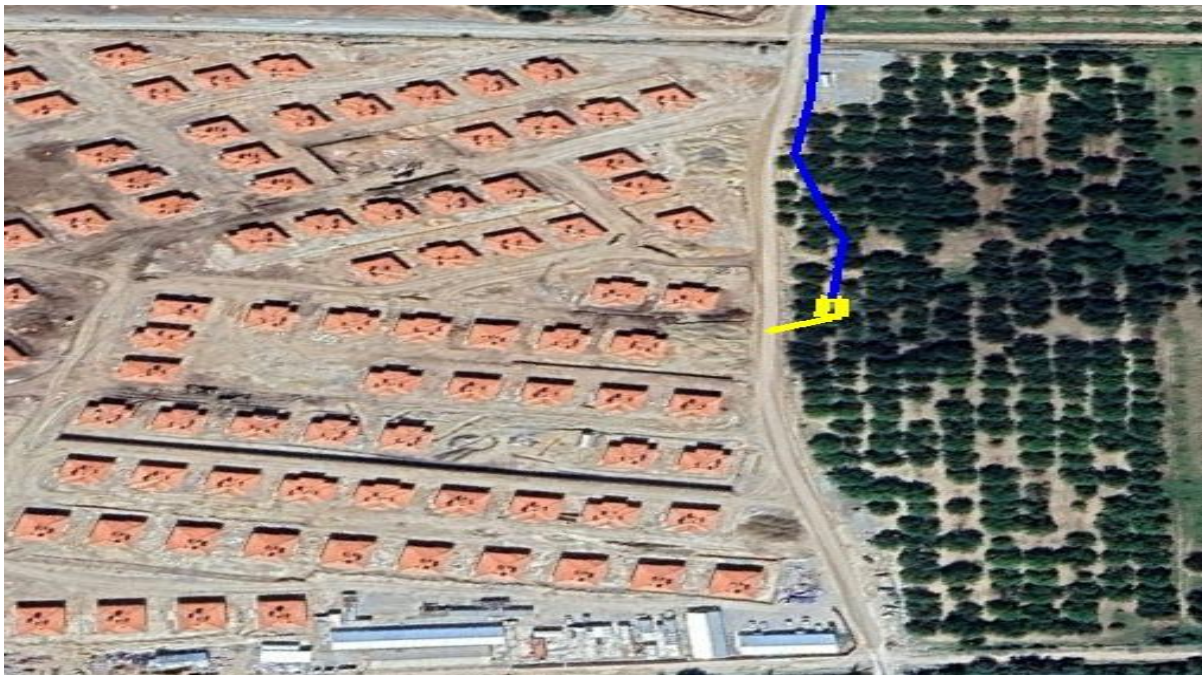
Figure-4 Wastewater Pumping Station Location on Google Earth
