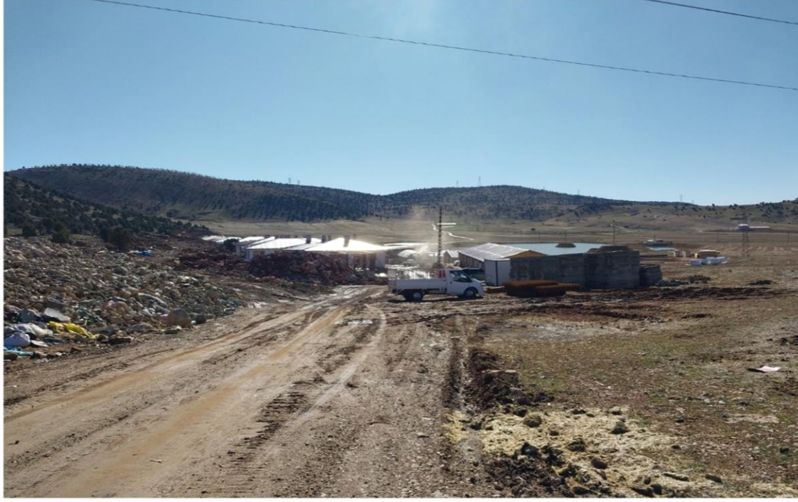
Photo 3: Karşıyaka (Fatih) TOKI Rural House Construction area next to the Parcel 168/100
