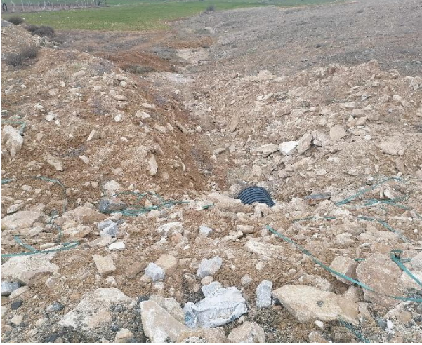
Photograph 44. Infrastructure Work (Piping)
