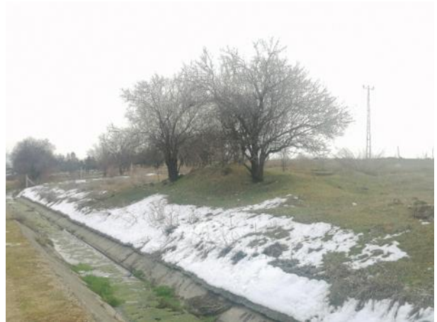
Photograph 12. Irrigation Channel and Trees
