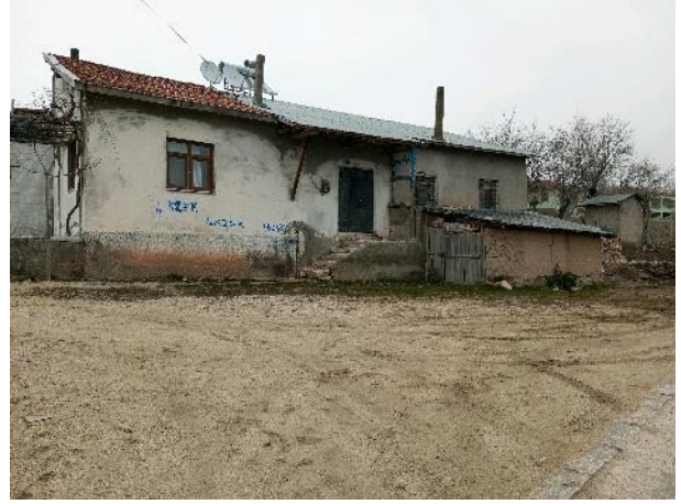
Photograph 56. General View of 102/38 Parcel-2
