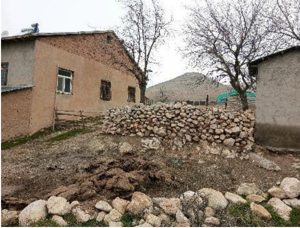
Photograph 57. General View of 102/38 Parcel-3 (adjacent house)
