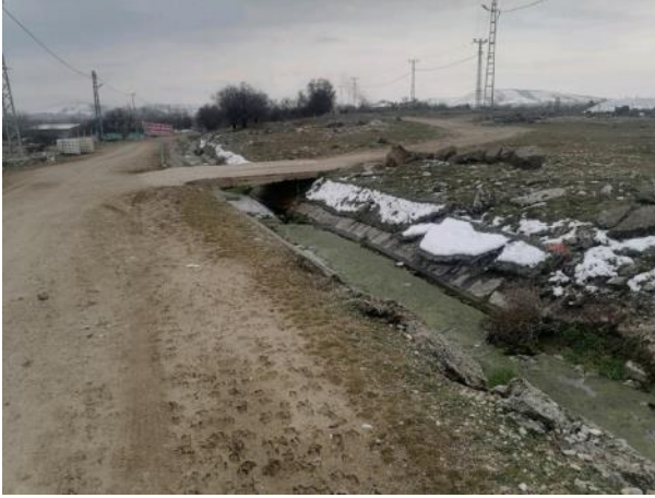
Photograph 7. Irrigation Channel at the Border of Parcels
