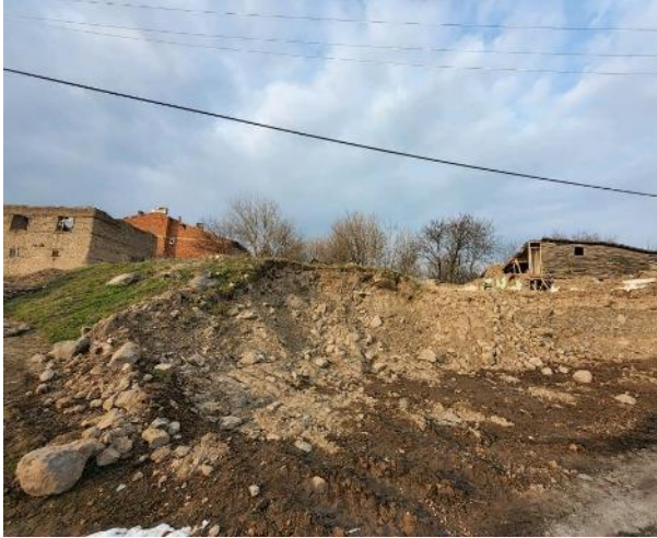
Photograph 19. General View of 160/21 Parcel-2
