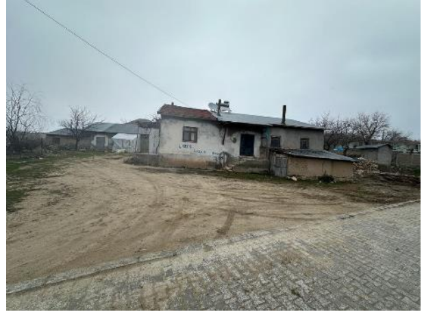
Photograph 58. General View of 102/38 Parcel-4 (directly connected to the access road)
