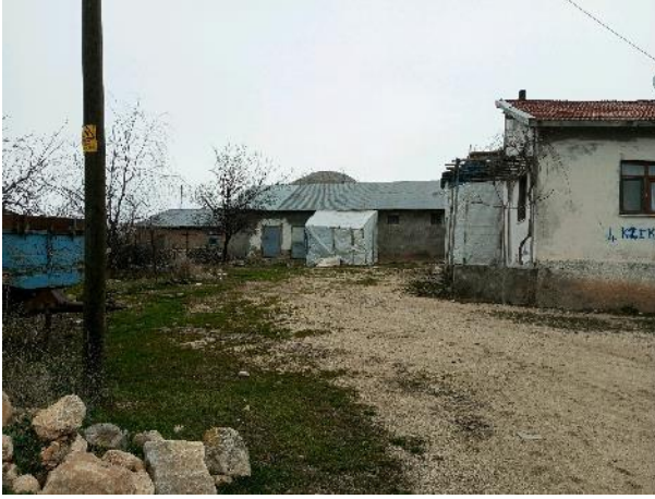
Photograph 55. General View of 102/38 Parcel-1
