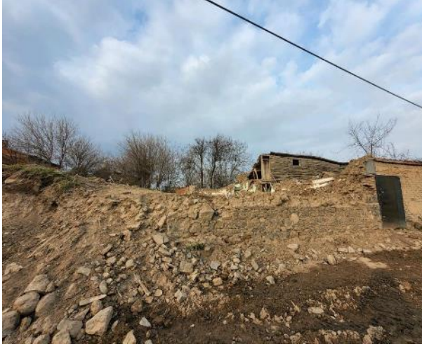
Photograph 17. General View of 160/21 Parcel-1
