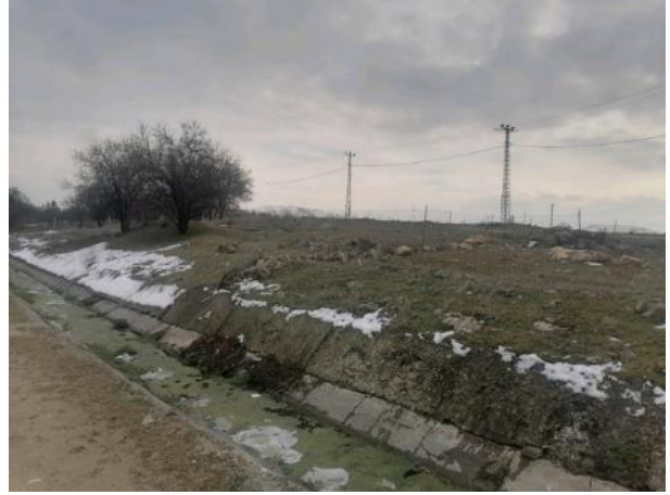
Photograph 8. Trees and Electric Transmission Line
