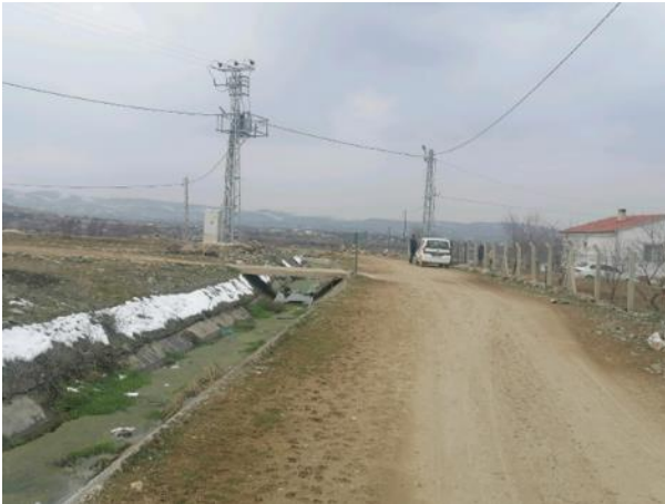
Photograph 11. Village Road and Irrigation Channel
