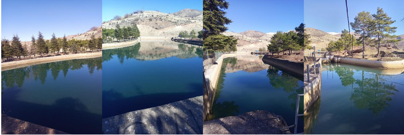
Photograph 9. General View from the HEP Pond
