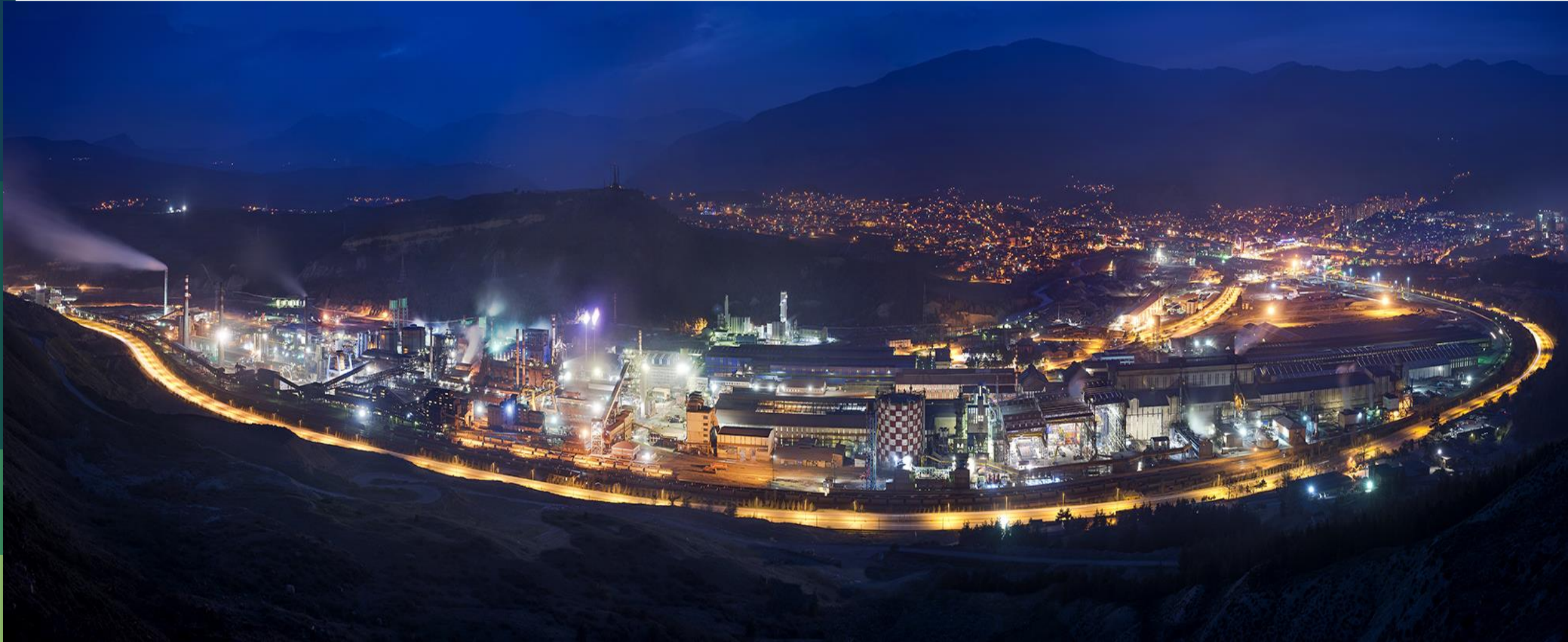
KARDEMIR (IRON&STEEL FACTORY)
