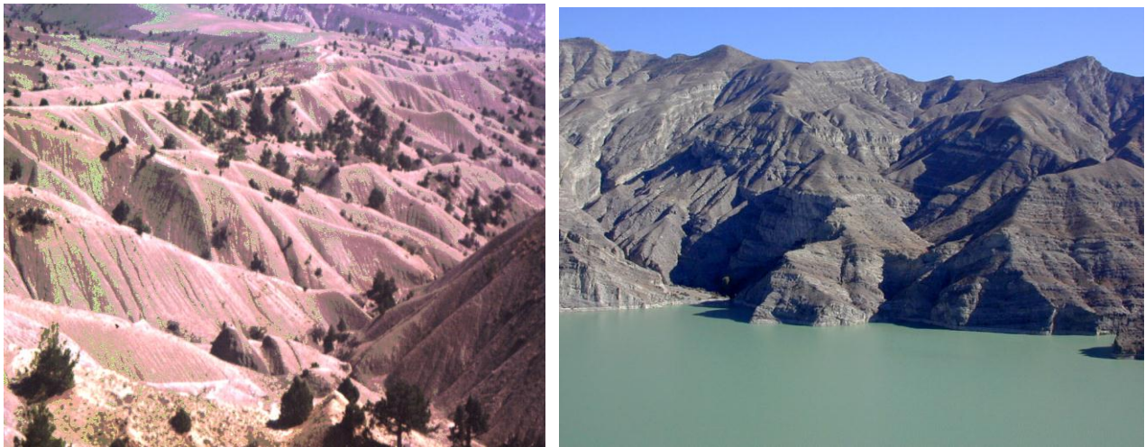
Figure 13. Sample areas where soil are being lost by severe erosion (AGM archive)
