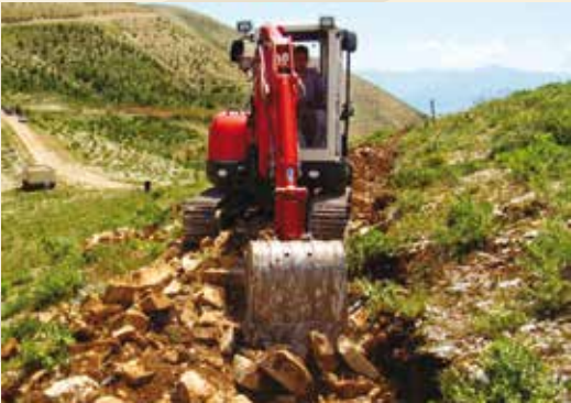
Terraces formed by crawler excavator
