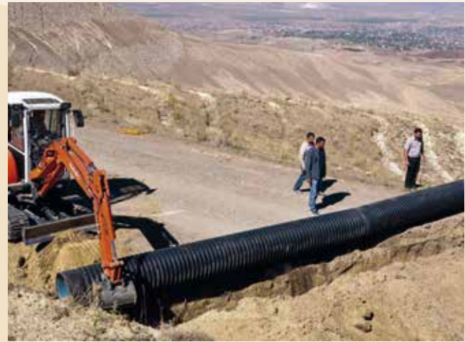
The corrugated Pipe was placed on the roads.
