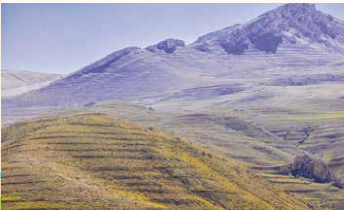
Slope Rehabilitation with Suitable Excavation Terrace. Terraced terraces are inclined in order to prevent soil movement.
