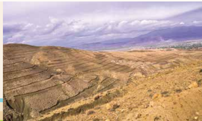
Slope Rehabilitation with Suitable Excavation Terrace. Terraced terraces are inclined in order to prevent soil movement.
