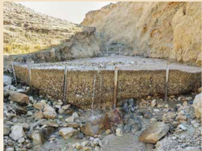
Systematic lattice wire barrier prevents soil transporting in gullies
