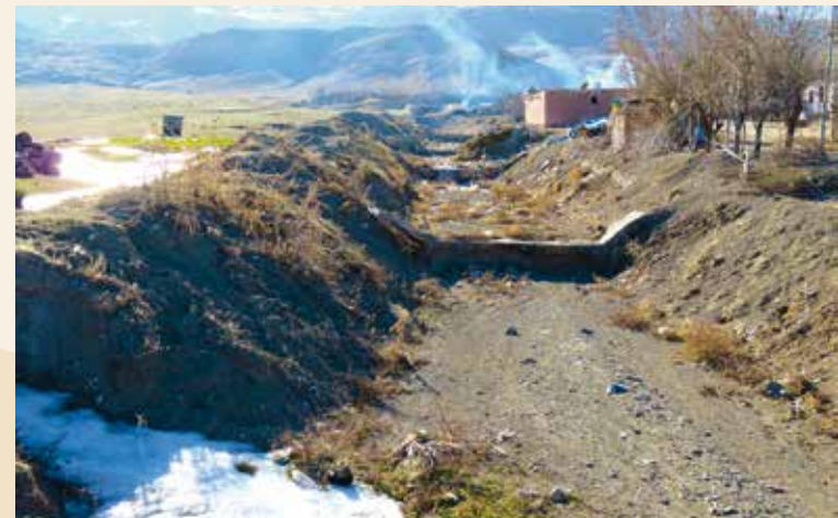
Ground sills and check dams built at regular intervals in a streambed/Watercourse
