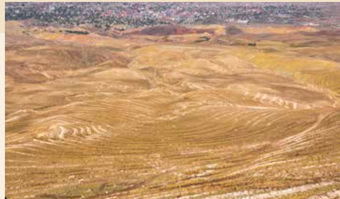
Slope Rehabilitation with Suitable Excavation Terrace. Terraced terraces are inclined in order to prevent soil movement.
