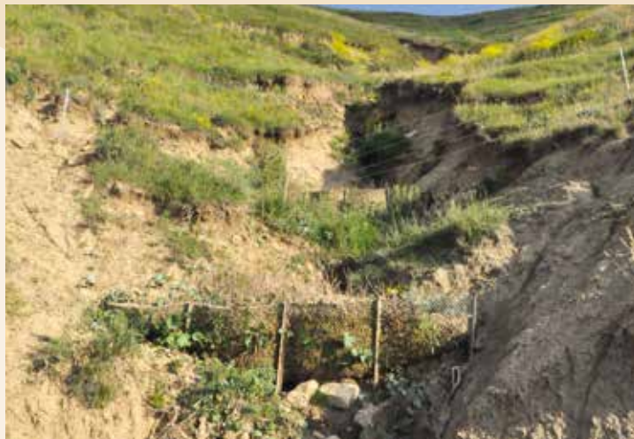
Systematic lattice wire barrier prevents soil transporting in gullies
