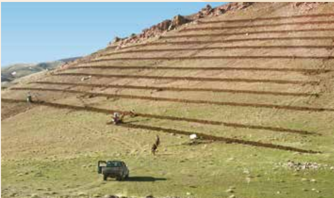
Slope Rehabilitation with Suitable Excavation Terrace. Terraced terraces are inclined in order to prevent soil movement.
