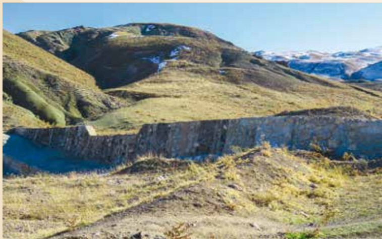
Ground sills and check dams built at regular intervals in a streambed/Watercourse
