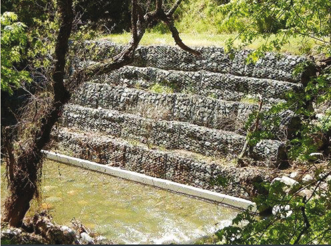
Gabion teras duvar
