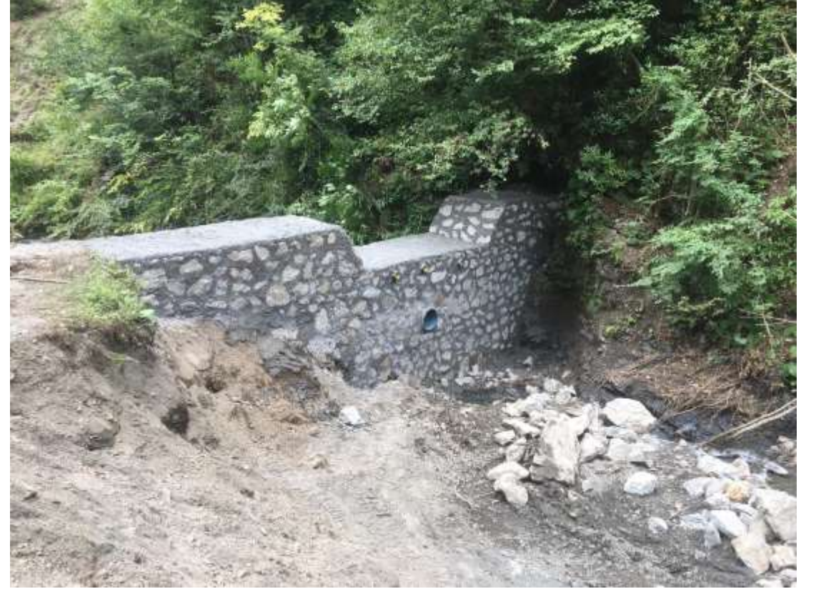
Ground Sills and Check Dams (Rize)
