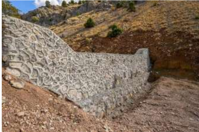
Ground Sills and Check Dams Built at Regular Intervals in a Streambed (Adana)
