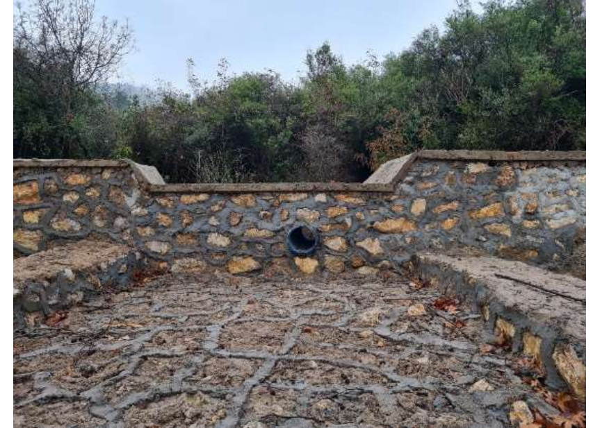
Ground Sills and Check Dams (Kisir - Aydın)
