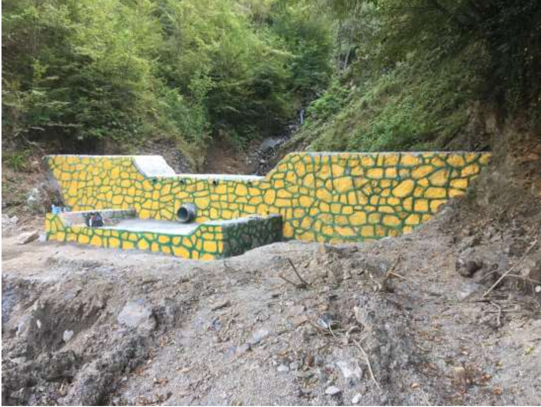
Ground Sills and Check Dams (Zonguldak)
