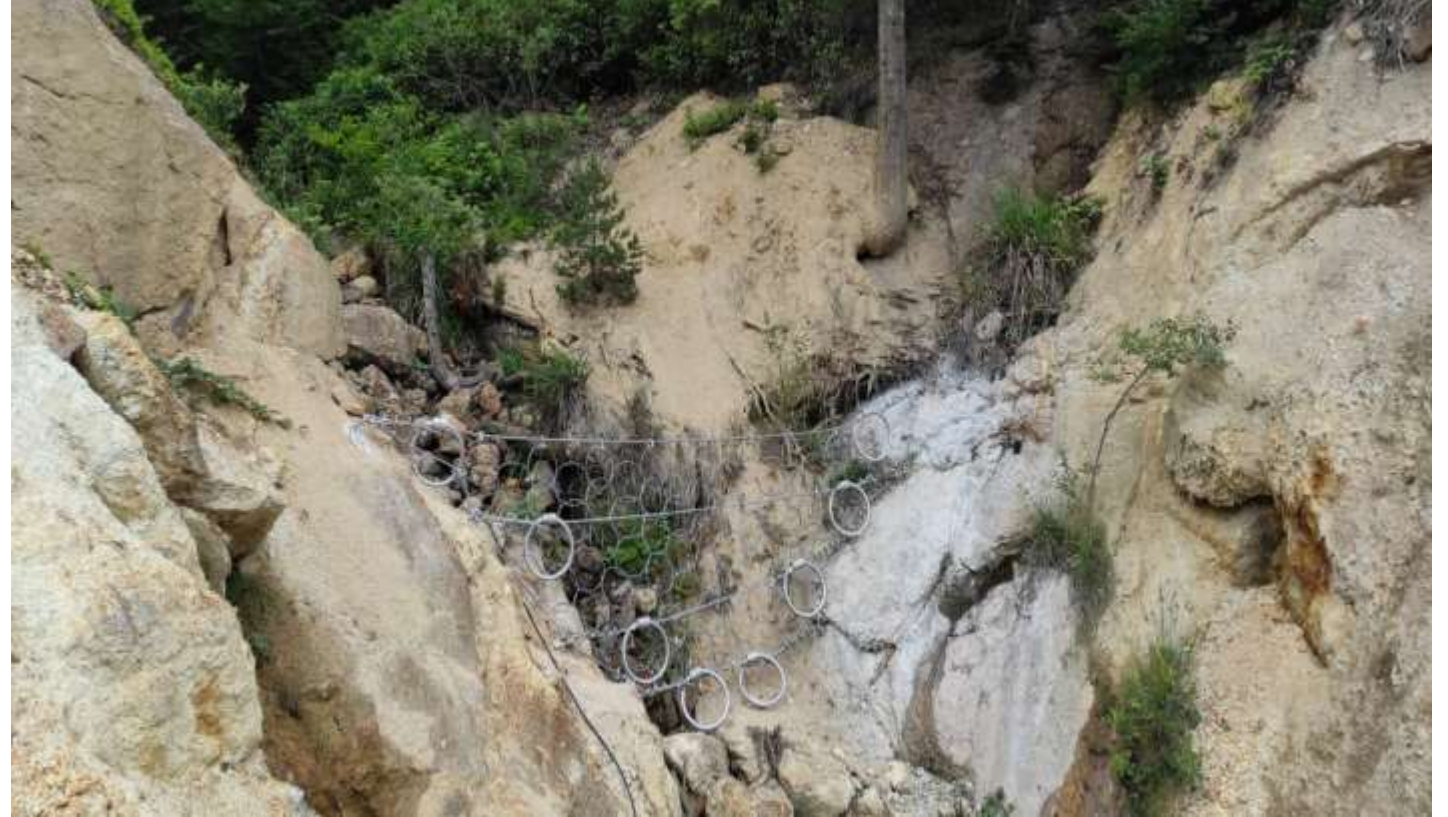
Steel-Mesh Debris Barrier (Trabzon)
