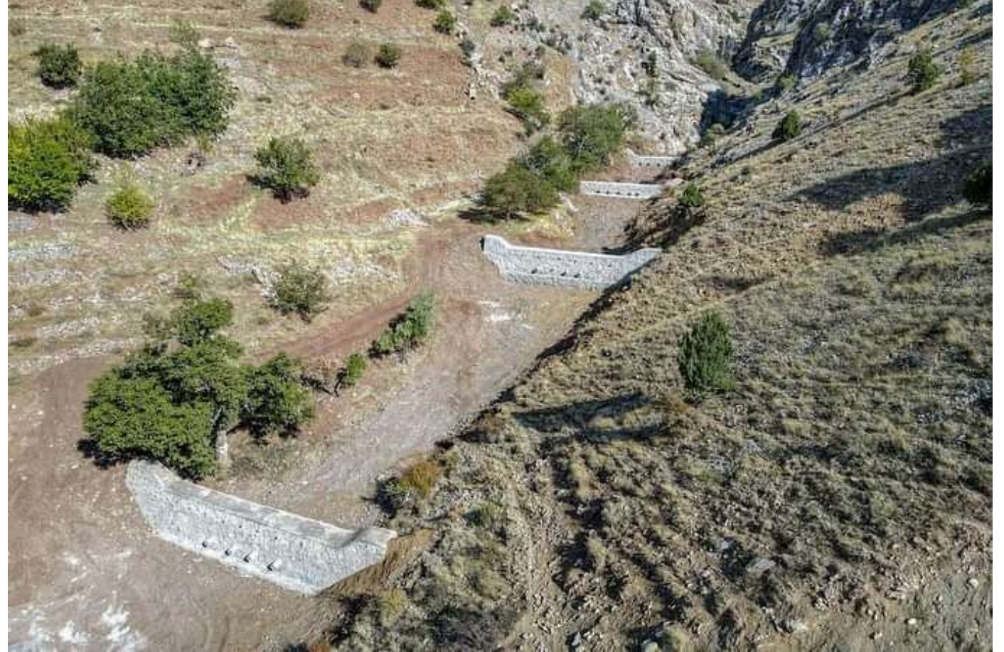
Ground Sills and Check Dams Built at Regular Intervals in a Streambed (Adana)
