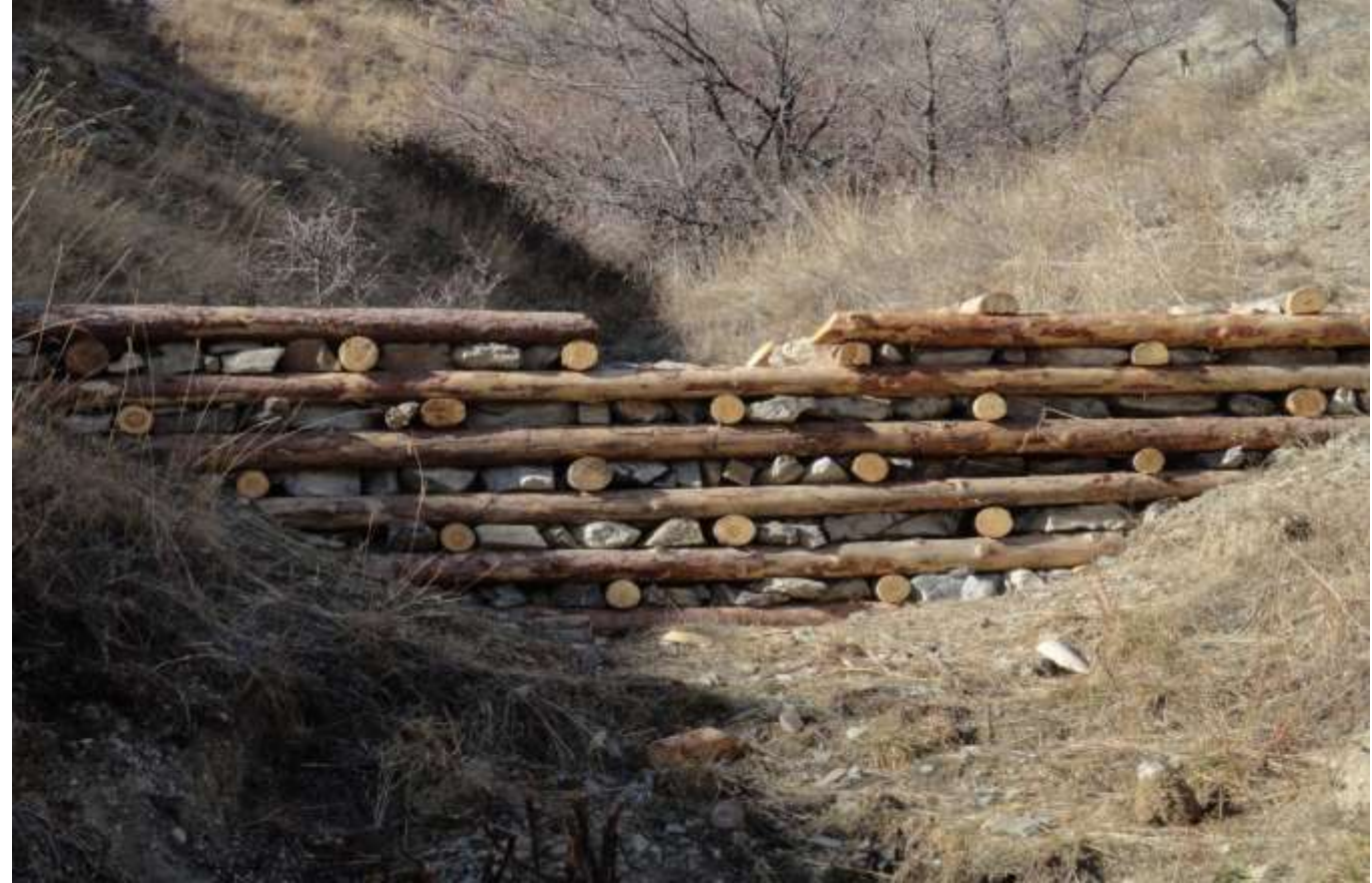
Wooden Check Dam (Ankara)
