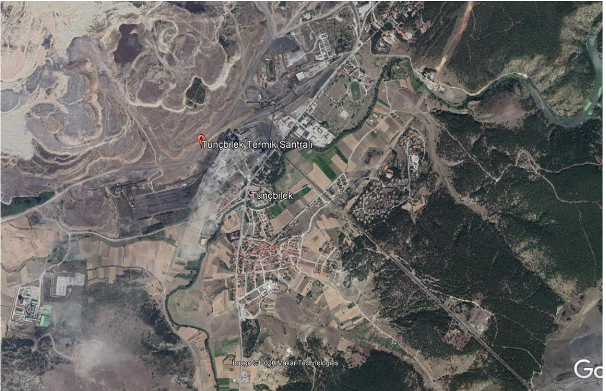
Harita C.4- Tunçbilek Termik Santrali 2020
