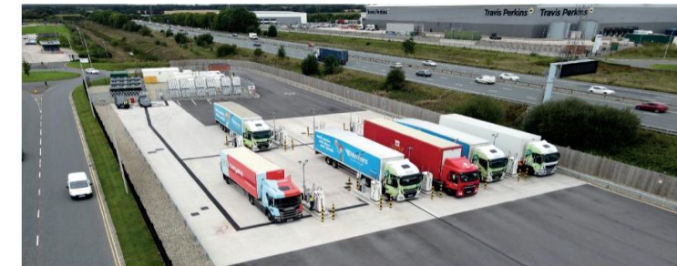
Figure 35. The large scale biomethane filling station in Warrington, UK. John Baldwin, CNG Services.
