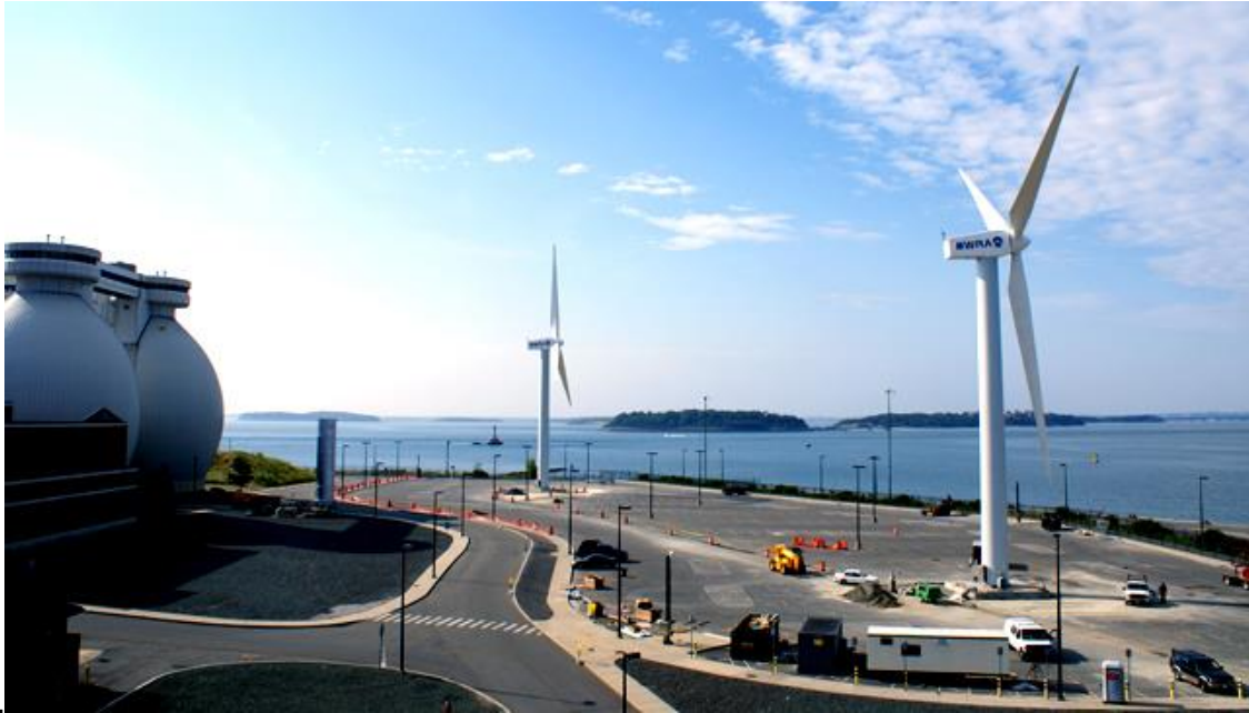
Şekil 3.24 ABD, Massachusetts - Deer Island Atıksu Arıtma Tesis (Massachusetts Water Resources Authority)
