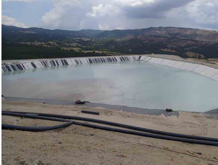
Photo 3- Organized storage facility for mining wastes
