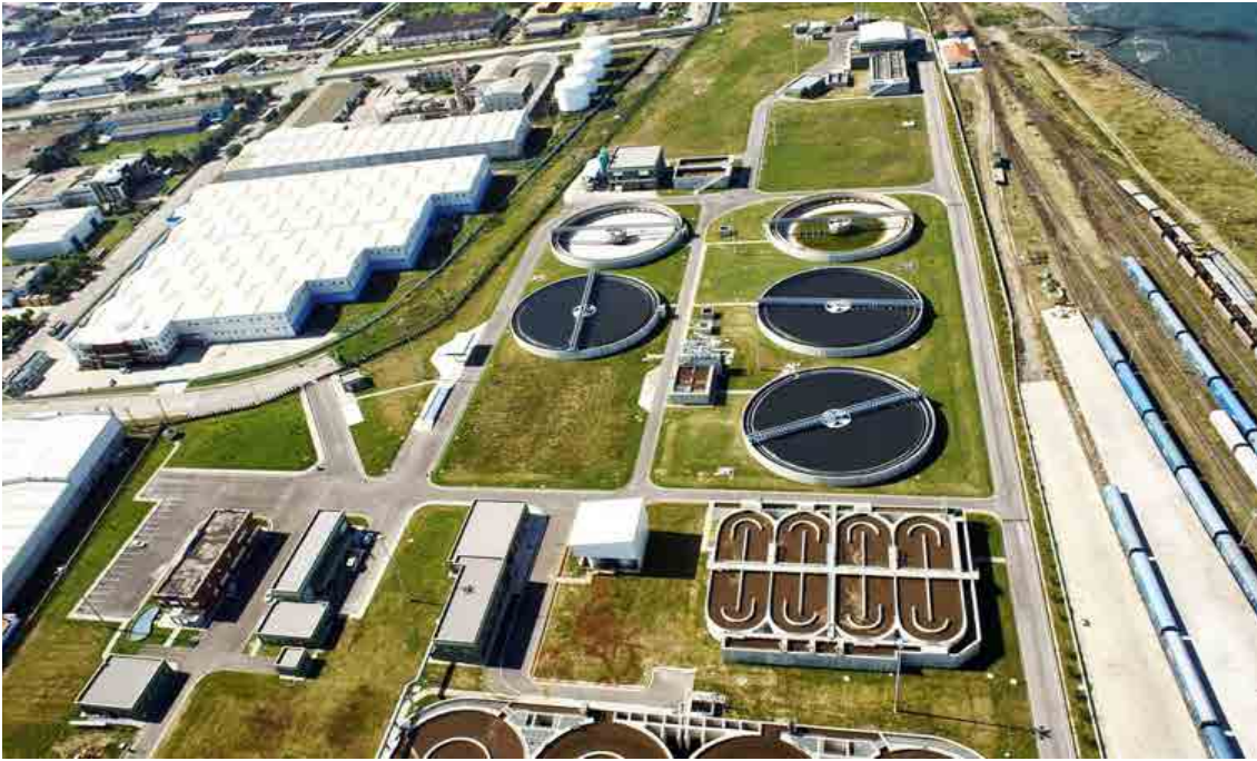
Photo 1– Samsun Doğu Waste Water Treatment Plant (Ministry of Environment and Urbanisation, 2016)
