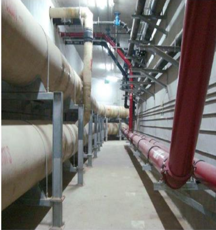
Figure 6.9. Example of wet utilities in a utility tunnel
