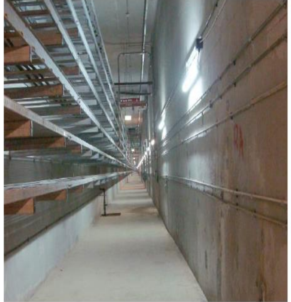
Figure 6.10. Example of dry utilities in a utility tunnel
